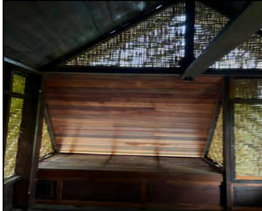
Figure 3: “Para Buang” at Rumah Kutai, Kompleks Pasir Salak
