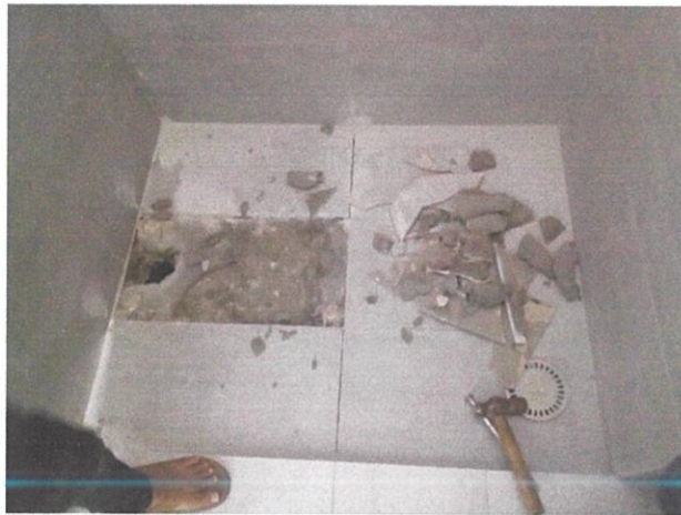
Figure 3.3.5 : Slab got a big hole.
