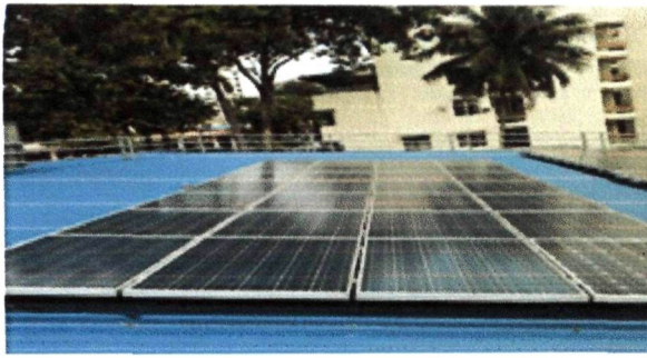
Fig. 2 Example of a 6.11 kWp GC system installed at GERC, UiTM Shah Alam, Selangor Darul Ehsan, Malaysia.
