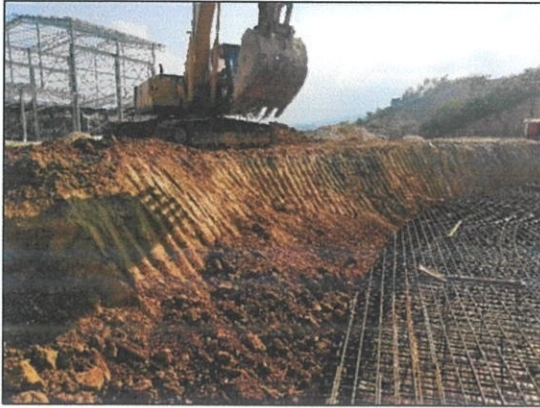
picture 3.9: excavate work
