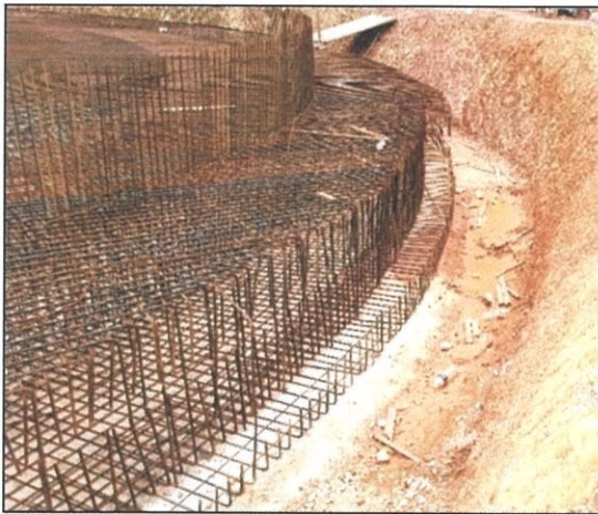
picture 3.11: adding steel reinforcement bar
