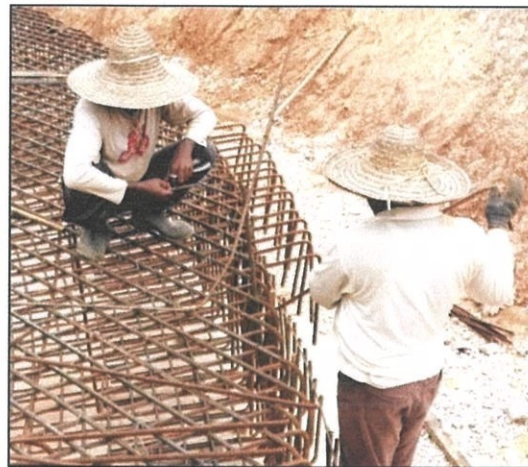
picture 3.12: adding steel reinforcement bar
