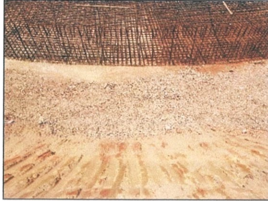
picture 3.10: pouring the crusher run
