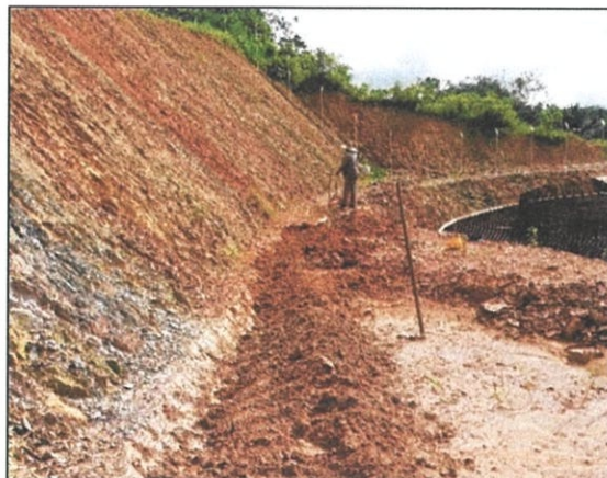
picture 3.5: built the temporary drain
