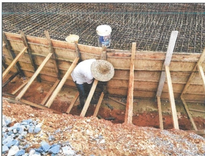
Picture 3.3: installing the formwork
