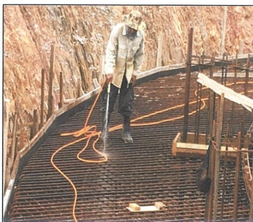
picture 3.6: cleaning the mud
