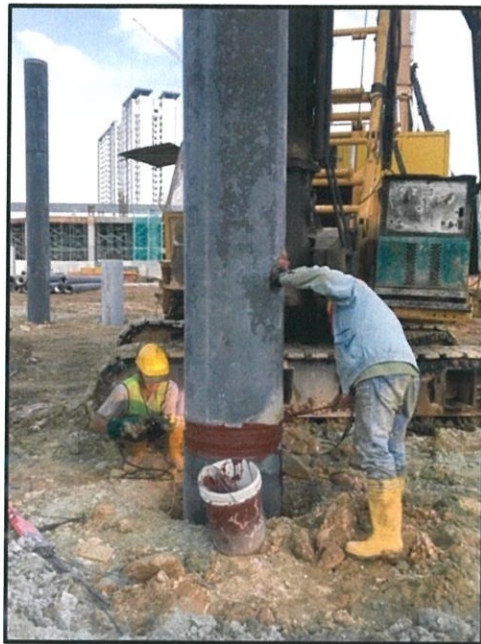
Figure 3.21: Coating is applied to cover the welded parts from rust
