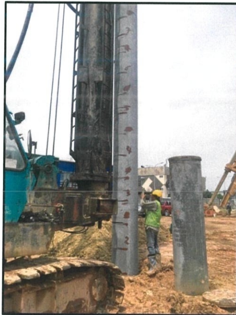
Figure 3.15: Pile assistant is checking the verticality
