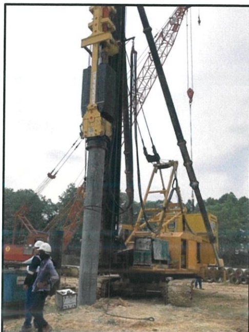
Figure 3.17: Mounted up the pile with the leader of pile machine
