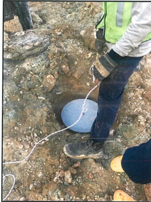
Figure 3.25: Closing the installed pile
