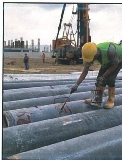
Figure 3.14: Marking the intervals in meters
