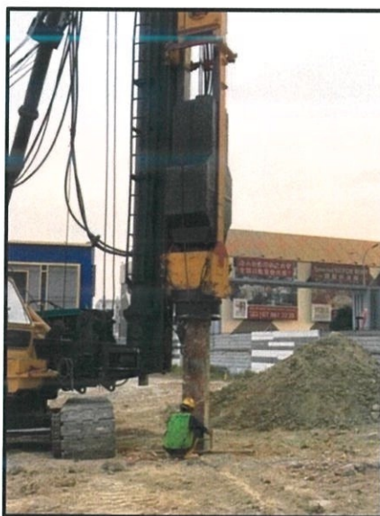
Figure 3.22: Taking the final set
