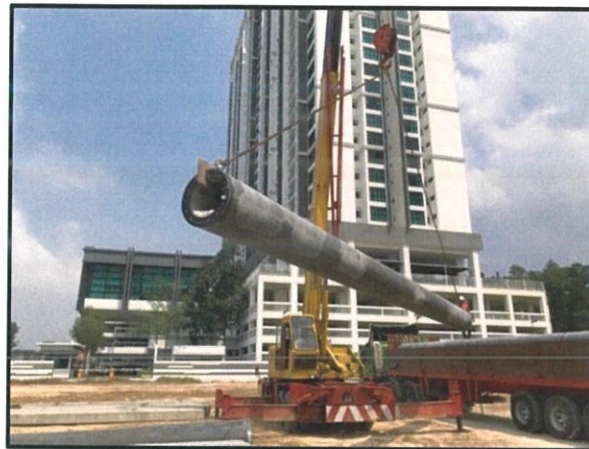
Figure 3.13: Transporting the spun pile onto a flat surface
