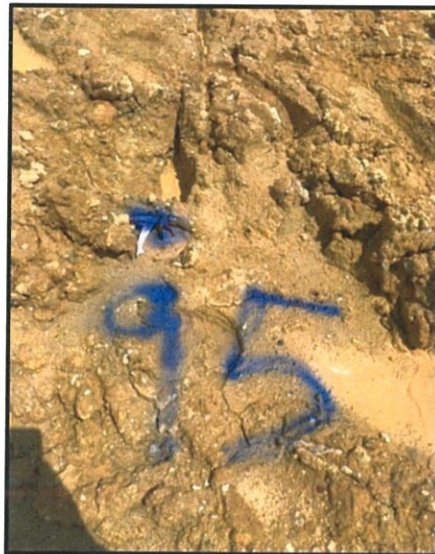
Figure 3.6: Peg the surveyed point and mark the point number
