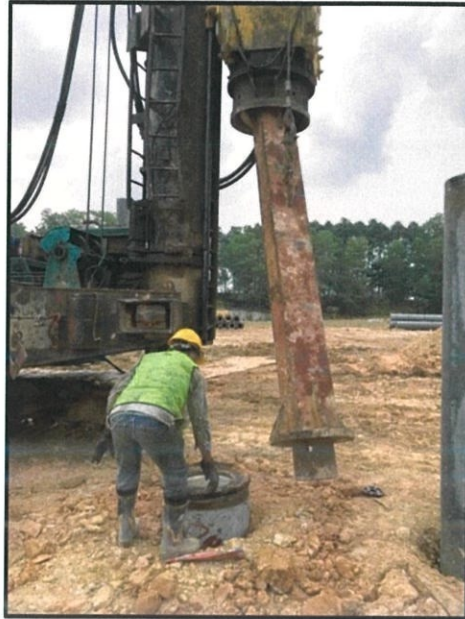
Figure 3.19: 2.5m to 3.0m dolly is used to get the final set
