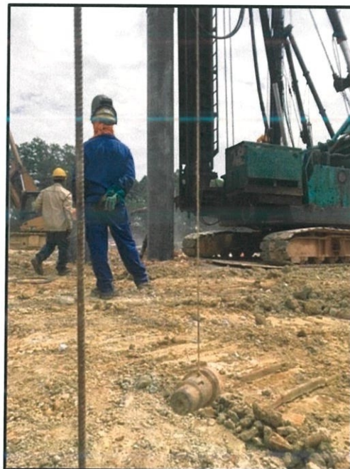
Figure 3.16: Verticality checking with plumb bob
