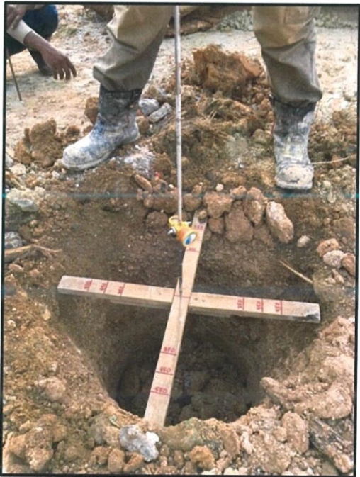
Figure 3.8: Checking the eccentricity with surveying equipment
