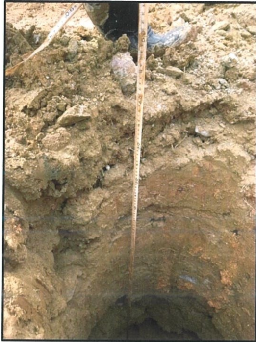
Figure 3.11: Checking the achieved pre-bore depth
