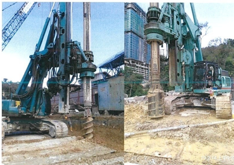
Figure 3.11 Setting Auger's Drilling Machine at Position
