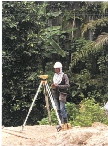
Figure 3.10 Setting Out by Surveyor
