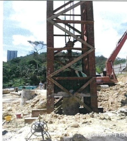
Pile Driving Analyzer Test (PDA TEST)
