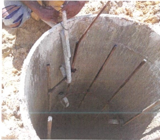
Figure 3.17 Position Reinforcement Bar using j-hook
