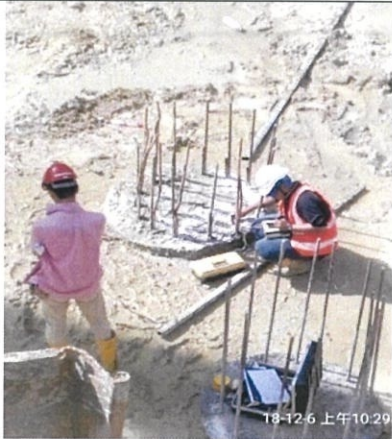
Pit Integrity Test (PIT)
