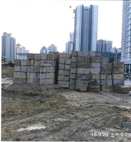
Maintain Load Test (MLT)
