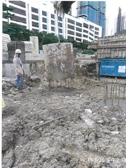
Figure 3.20 Remove of Temporary Casing
