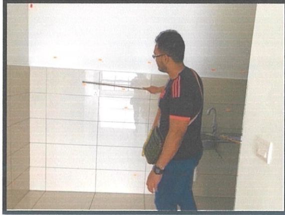
Figure 3.4 Supervisor check the hollow tiles put sticker by the owner
