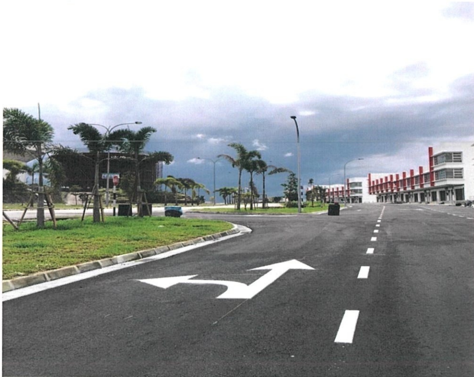
Figure 2.10 – Shows the road marking has been laid with paint added with filling & glass beads for high shine
