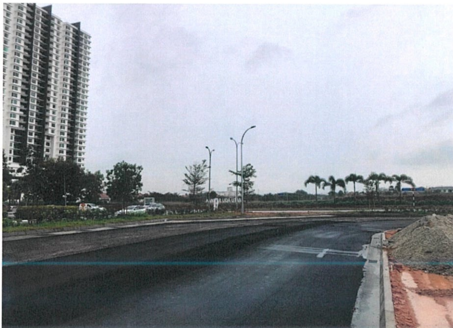
Figure 2.6 – Shows the road has been coated with tack coat RS1K
