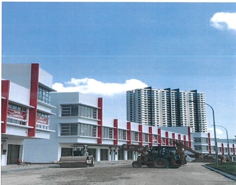
Figure 2.3 – Shows the Neuvo Centro 2 construction site
