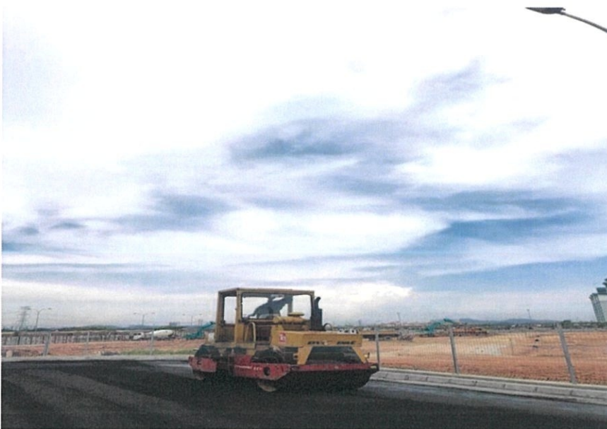
Figure 2.9 - Shows the roller compacting the premix to the right compaction
