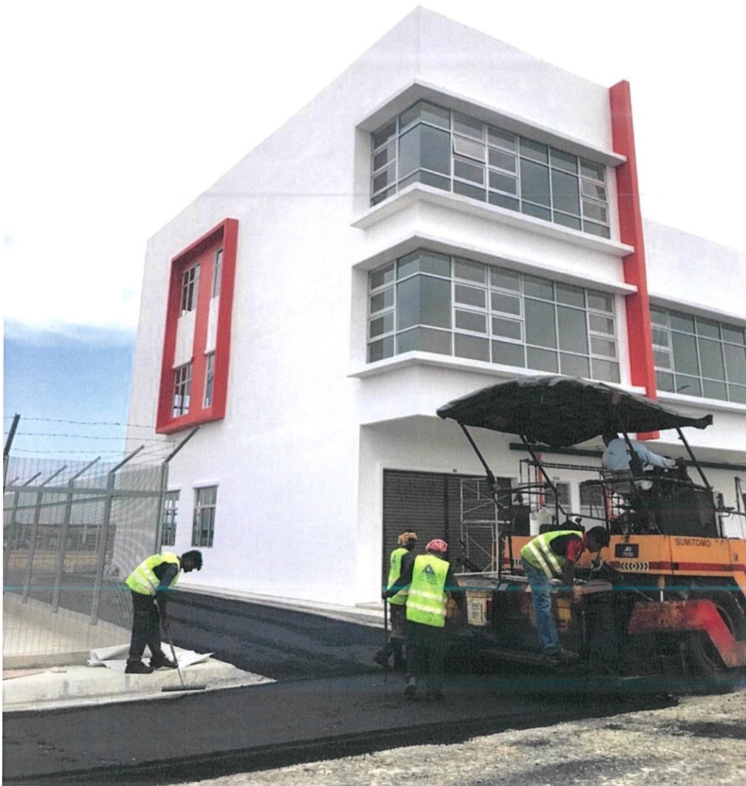
Figure 2.16 – Shows the premix being laid for the Neuvo Centro 2
