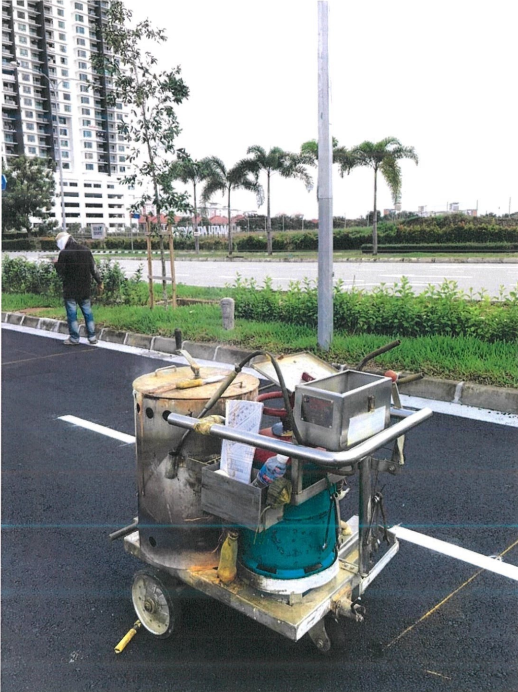
Figure 2.15 – Shows the road marking equipment with paint and glass beads
