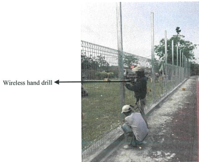
Figure 3.10 Tighten the bolt and nut.
