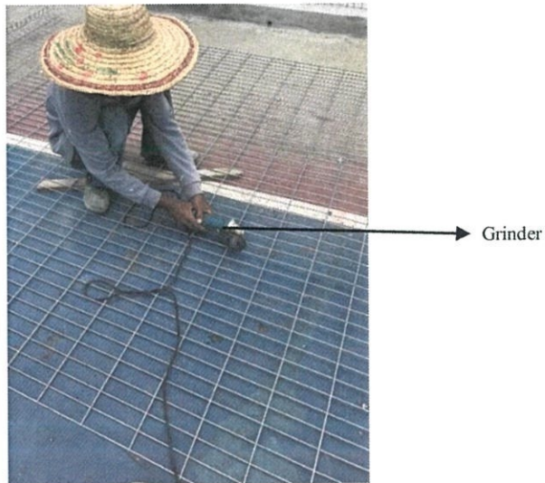
Figure 3.12 Cutting the fences.
