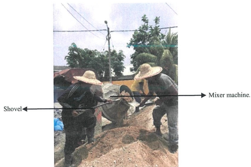
Figure 3.5 Concrete mixing work.
