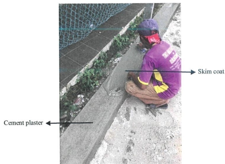
Figure 3.8 Plastering works.
