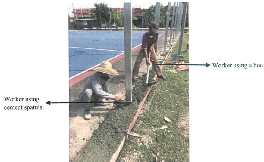
Figure 3.6 Concrete spread into formworks.
