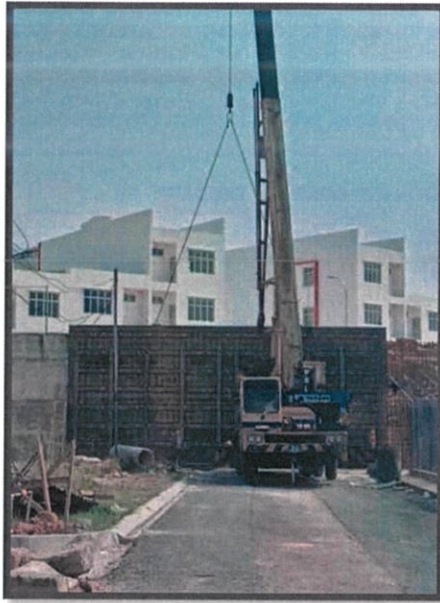
Figure 35: Steel formwork lifted by using the crane.
