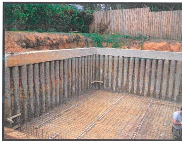
Figure 23: Piling wall
