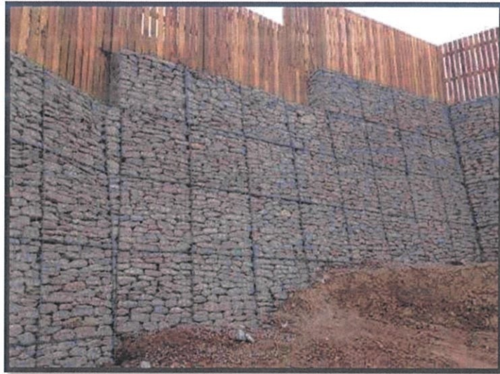
Figure 17: Gabion retaining wall.
