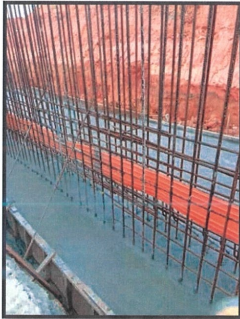
Figure 32: Final look of the strip footing concrete works.
