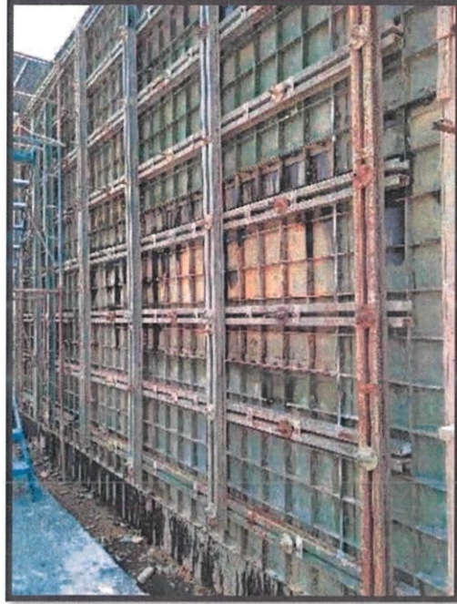
Figure 40: Steel formwork at 10.8 m distance post – concrete.
