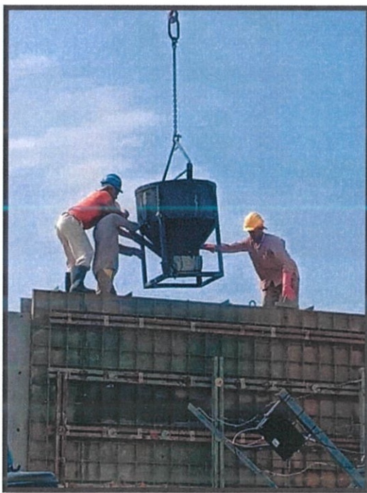
Figure 39: Concrete, grade 30 cast into the steel formwork.
