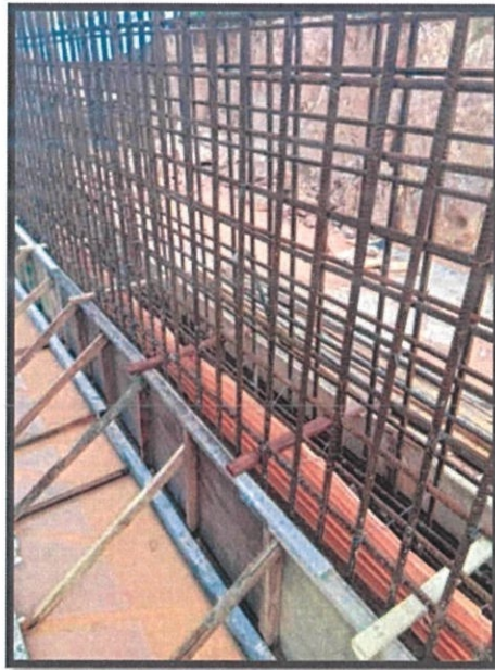
Figure 27: Water stops has been installed.
