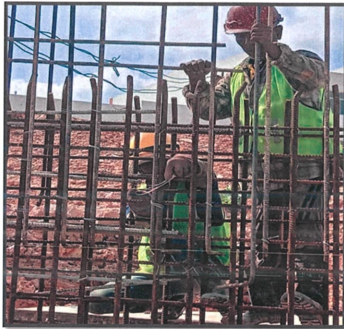
Figure 25: Installation of reinforcement bar at wall structures.
