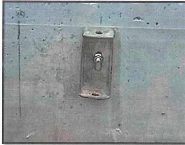
Figure 33: Double C-channel support.
