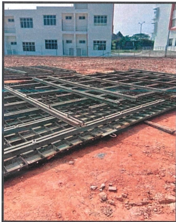
Figure 34: Steel formwork arrived, front and back.
