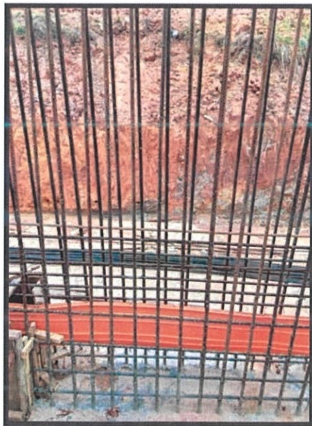
Figure 28: PVC water stops (orange); 12.0 m x 0.30 m.
