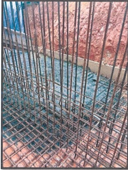
Figure 31: Strip footing concrete works.
