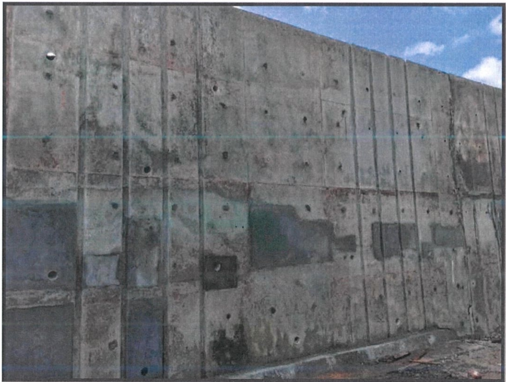
Figure 41: After concrete process.
