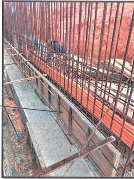
Figure 30: Tapered side of wall formwork installed.
