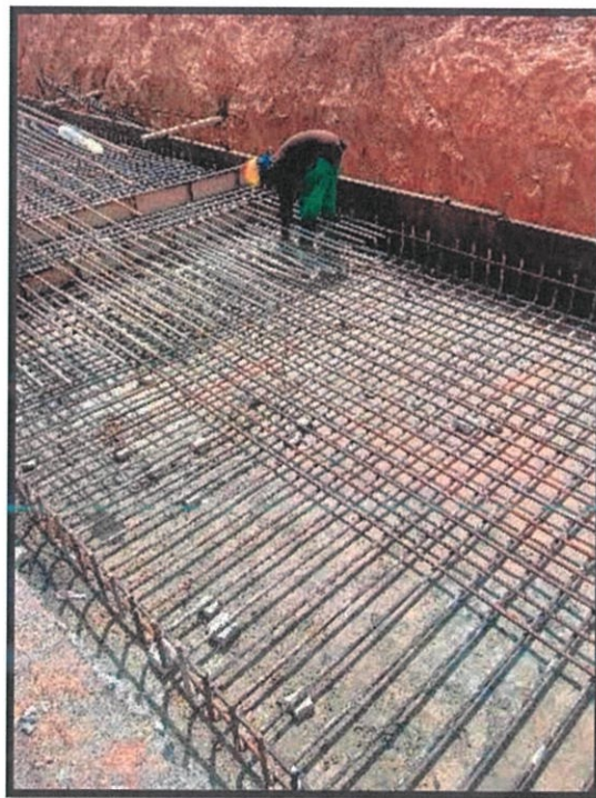
Figure 26: Reinforcement bar installed at strip footing.
