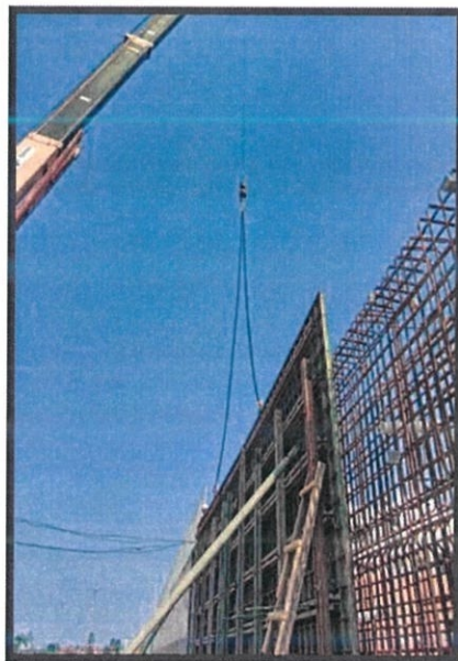
Figure 36: Steel formwork laid on the required position.
