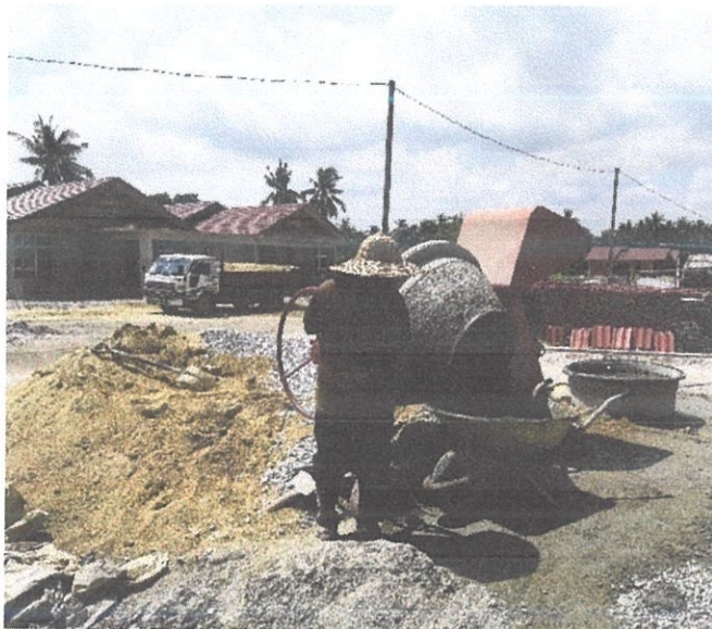
Figure 3.11: Concrete Mixing by Machine
