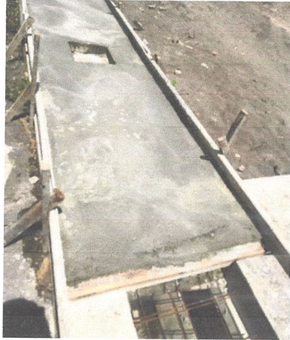
Figure 3.12: Concrete Poured into the Formwork case
