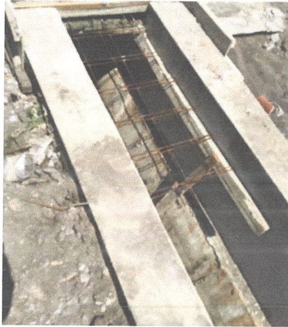
Figure 3.10: Installation Rebar
