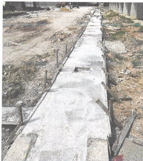
Figure 3.13: Concrete Hardened After Several Days
