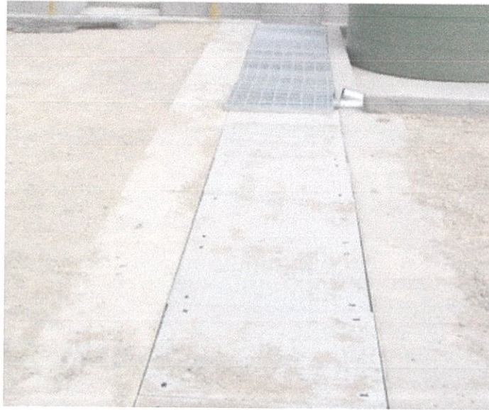
Figure 1.2: Steel Crossing Plate
