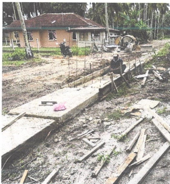
Figure 3.9: Reinforced Bar Installation
