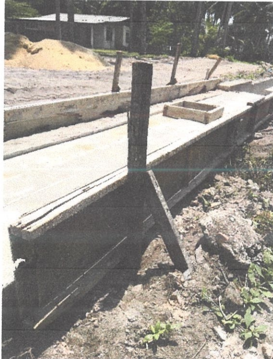
Figure 3.7: The Complete installation of Formwork Case
