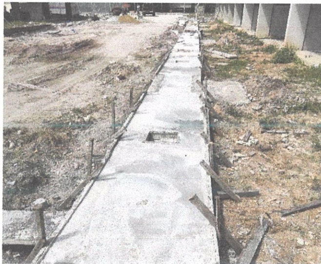
Figure 1.1: Concrete Crossing Slab
