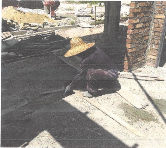
Figure 3.5: Making Formwork Case
