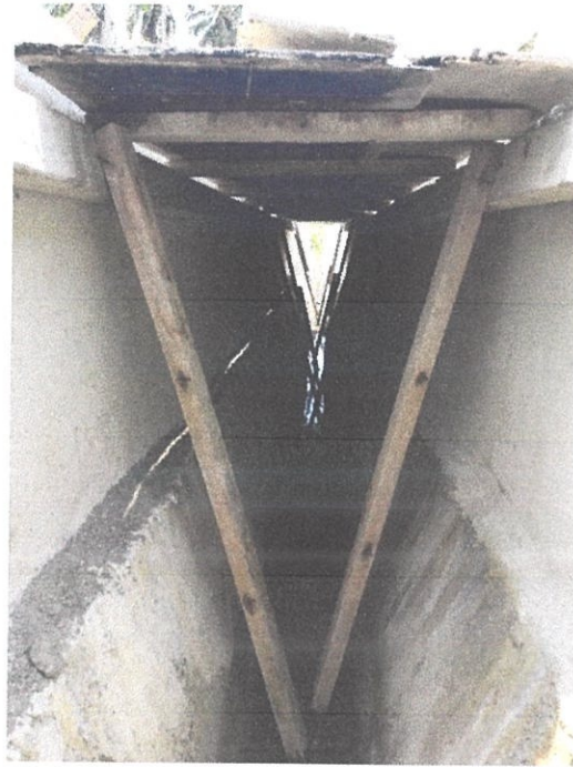
Figure 3.8: Formwork Stand
