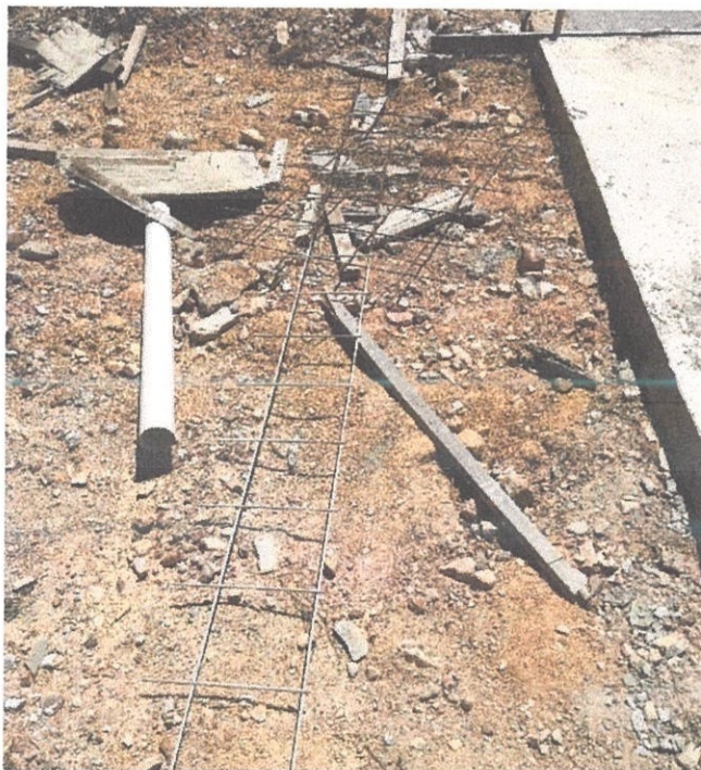
Figure 3.6: Preparation for Reinforced Bar
