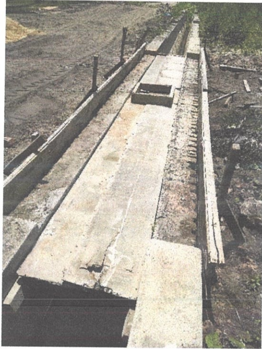
Figure 3.6: Installation of Formwork Case
