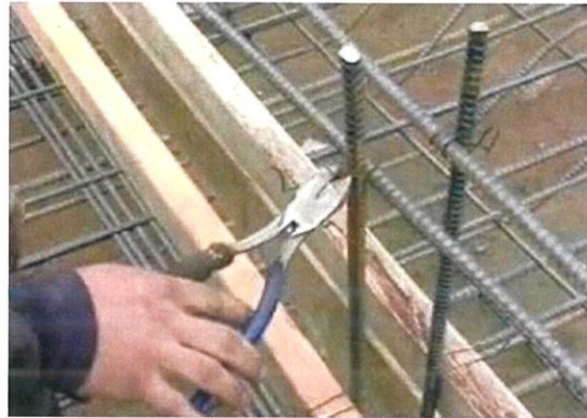
Figure 3.13: Tie the Reinforcement
