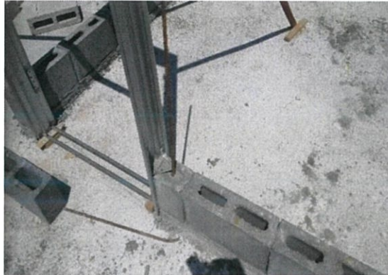
Figure 3.11: Construct Besides the Door Frame
