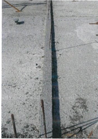
Figure 3.9: Completed of Kicker
