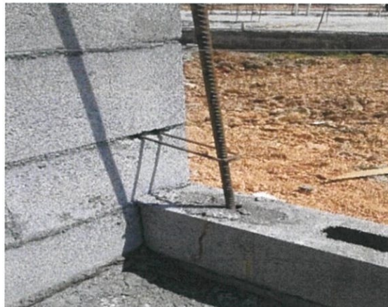
Figure 3.12: Construct at the Joint of Wall
