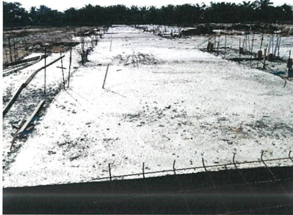
Figure 3.7: Floor completely screed
