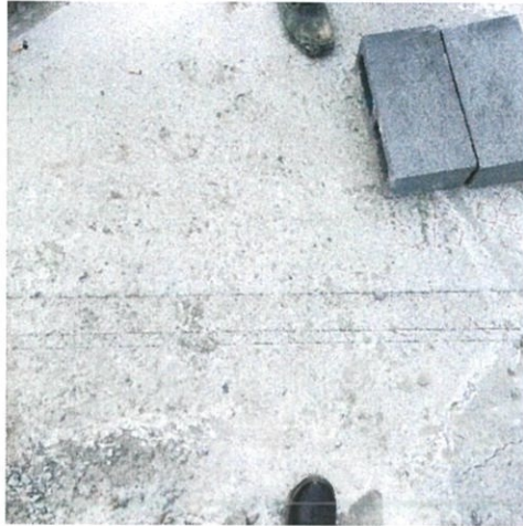
Figure 3.6: Mark from Setting Out by Surveyor
