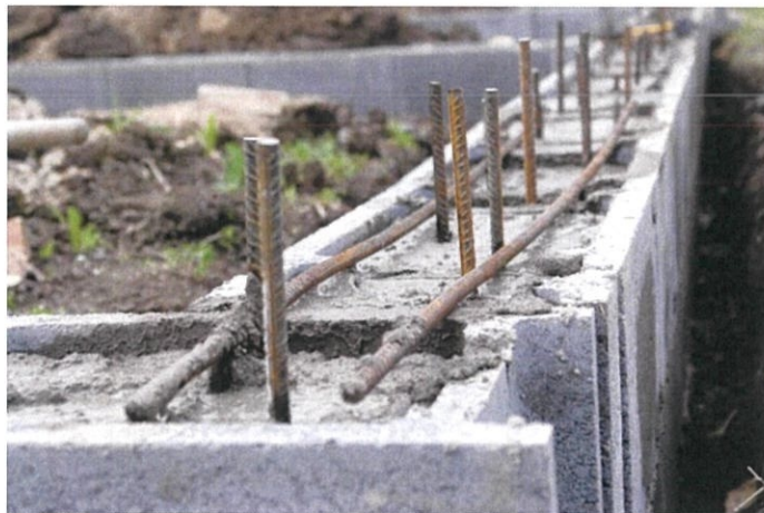
Figure 3.4: Block Infill with Grouting
