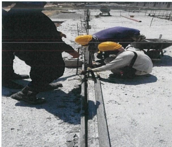
Figure 3.8: Lay Lean Concrete
