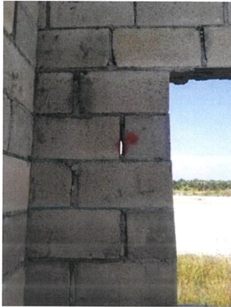
Figure 3.26: Hole Between the Block
