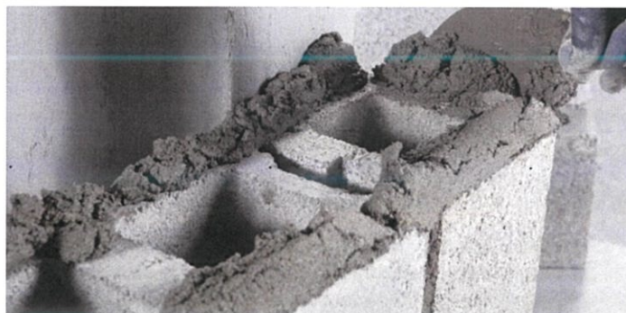
Figure 3.5: Mortar Being Placed Between Blocks
