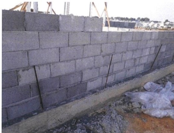
Figure 3.25: Placement of Reinforcement
