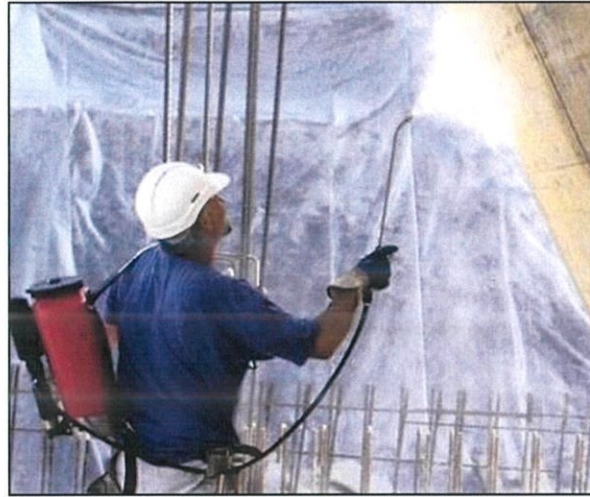
Figure 3.9 Spraying of releasing agent
