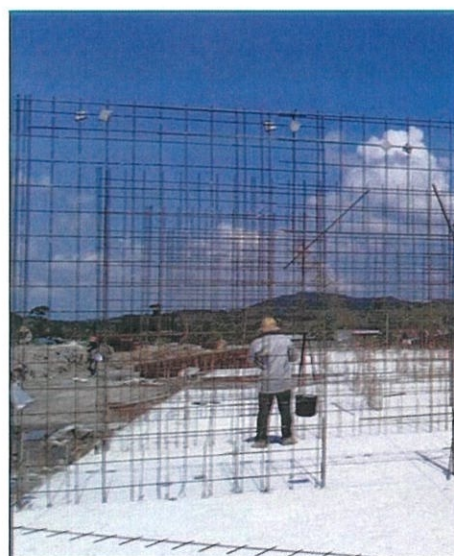
Figure 3.3 Erected wall rebar
