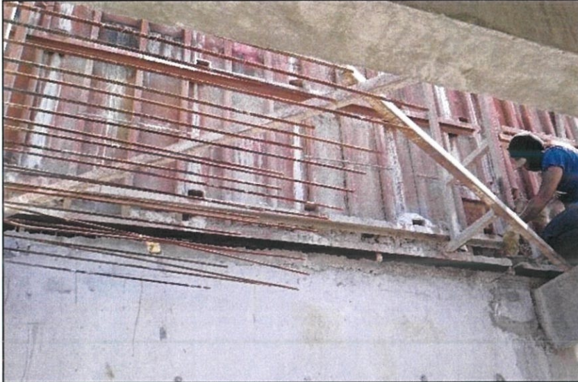
Figure 3.6 Steel formwork panel next to a stairwell opening
