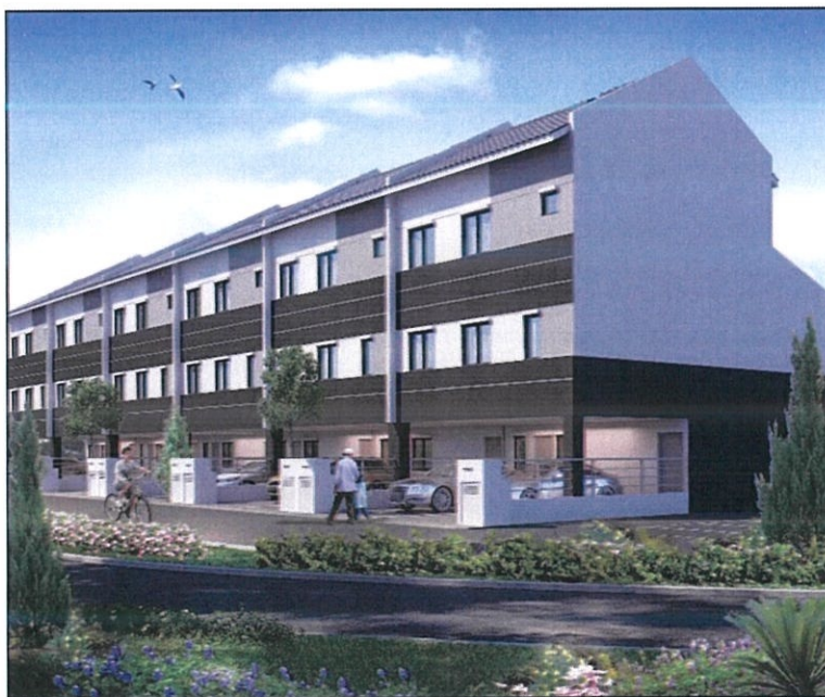
Figure 3.1 Illustration of completed construction
