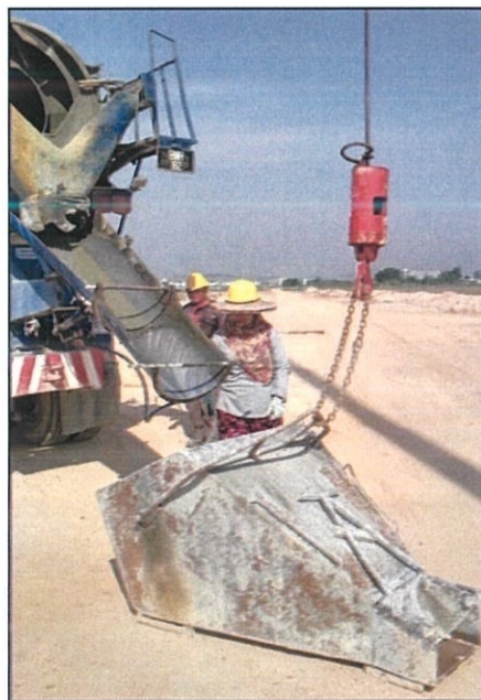
Figure 3.10 Mixer truck pouring concrete into bucket
