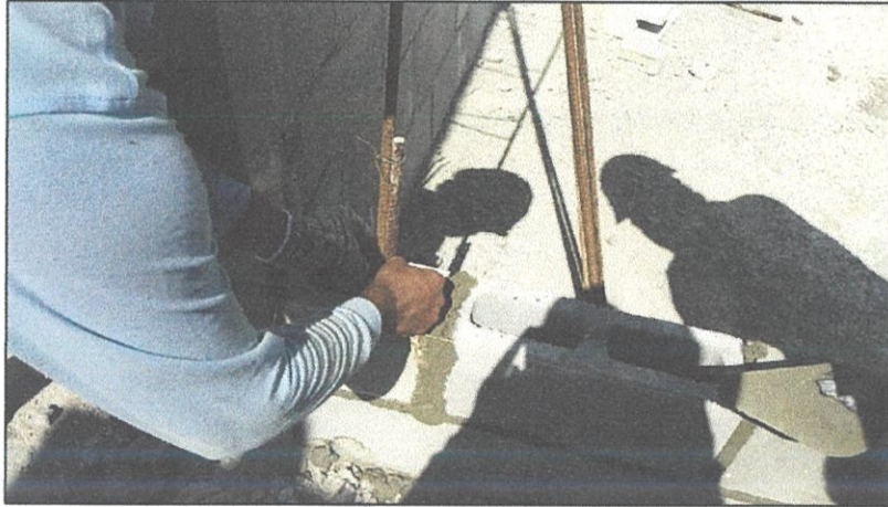
Figure 3.3.9 Installation of the connection of starter bar
