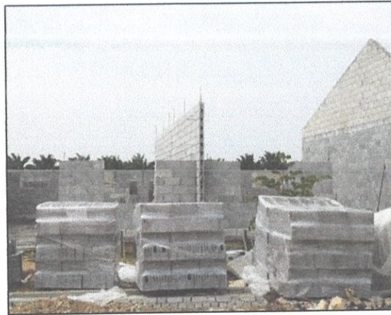
Figure 3.3.5 Place Construction Material at the Nearest Workplace
