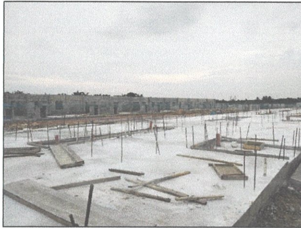
Figure 3.3.8 Area has to be cleaned before starting of work
