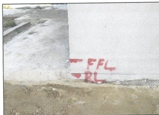
Figure 3.3.4 Marking of FFL and RL
