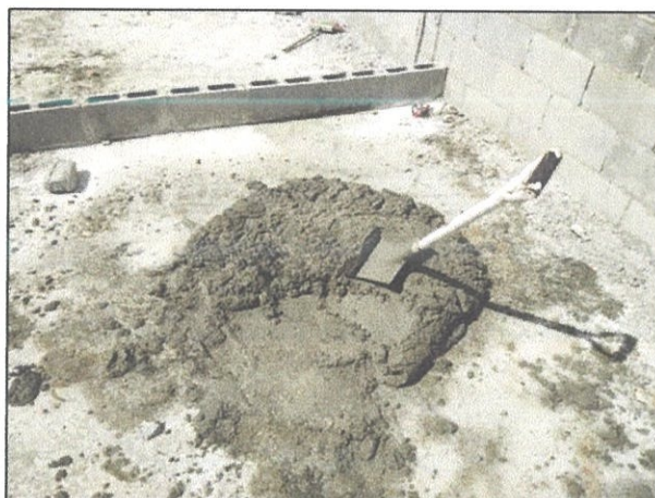
Figure 3.3.7 Mortar is ready to use
