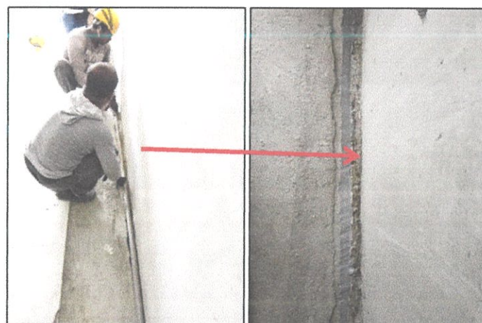
Figure 3.3.22 Process of expansion join at site
