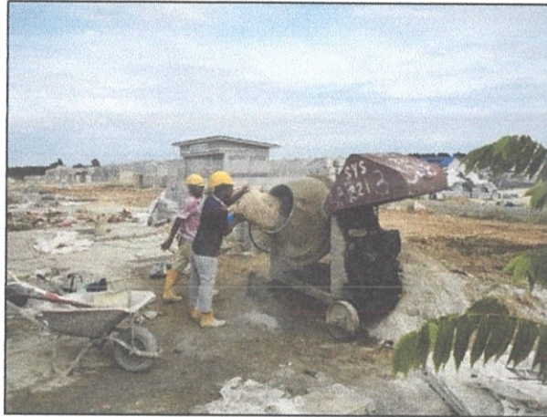
Figure 3.3.6 Subcontractor Prepare the Mixture of Mortar
