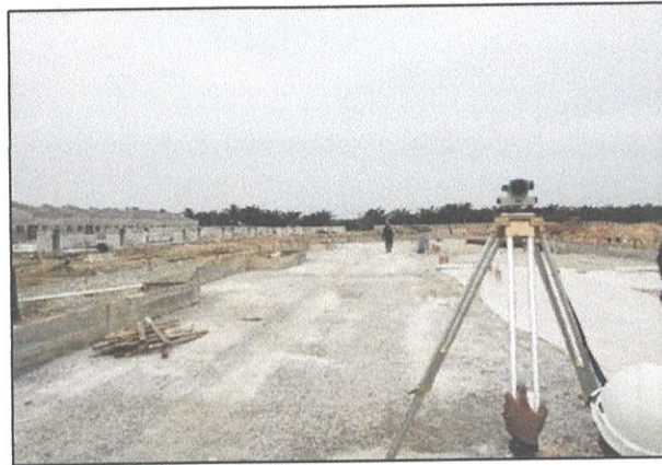
Figure 3.3.3 Setting Out and Marking of level
