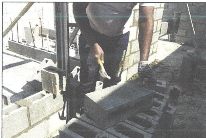
Figure 3.3.11 Marking the block in the required dimension before cutting it
