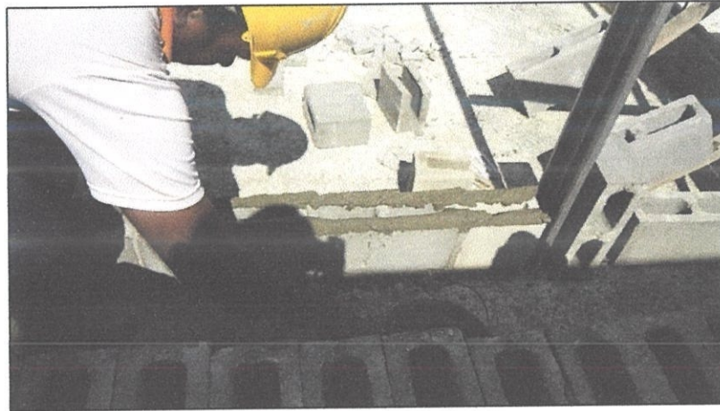
Figure 3.3.12 Mortar joint
