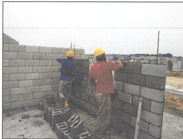
Figure 3.3.10 Laying of block wall
