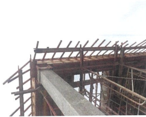
Figure 3.7 Side walls and beam soffits have been installed
