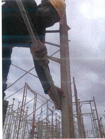
Figure 3.9 Cross bracing locking
