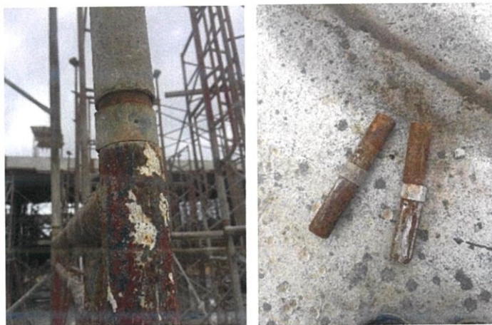
Figure 3.10 Fixing the joint pin into the scaffold frame
