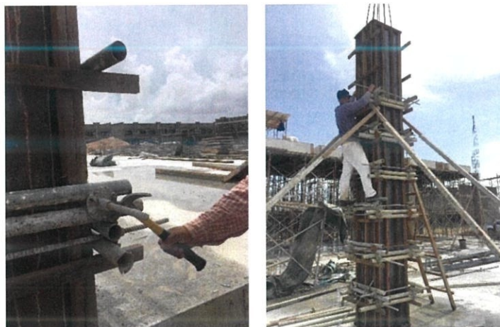
Figure 3.6 Column formwork clamping using tie rods and clamps
