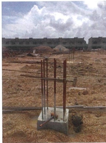
Figure 3.3 Column reinforcement bar checking
