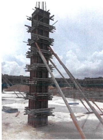
Figure 3.5 Column formwork is propped on both sides
