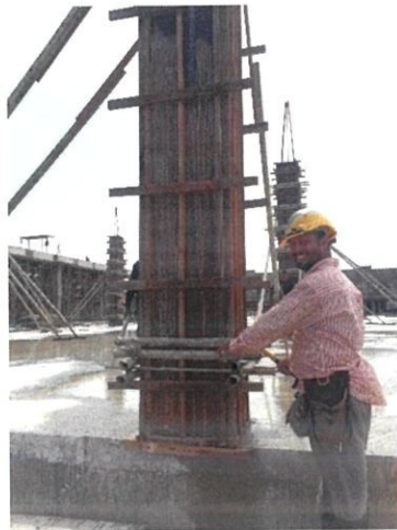
Figure 3.4 Constructing formwork
