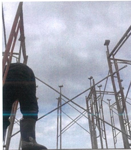
Figure 3.8 Scaffold frame installation
