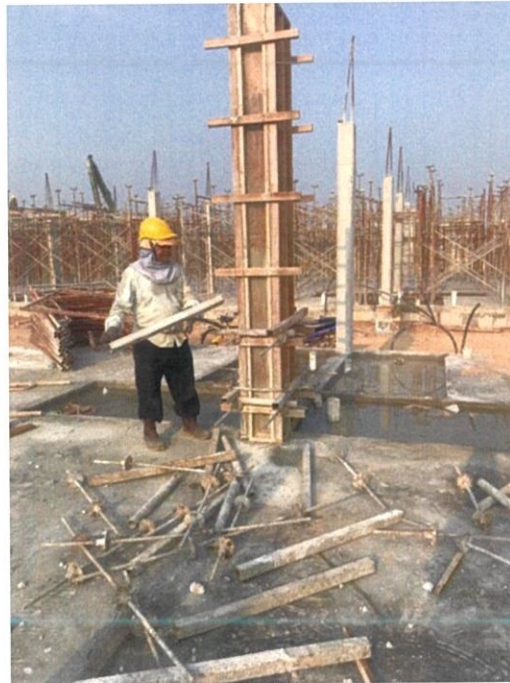
Figure 3.12 Column formwork dismantling process
