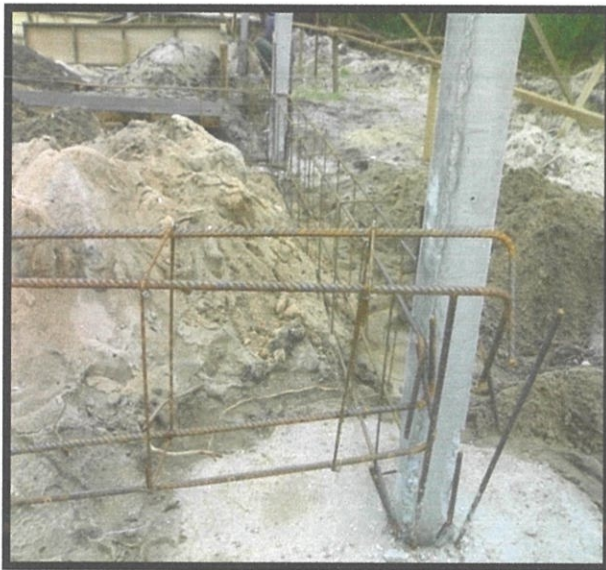
Figure 1.10 Reinforcement bar placement
