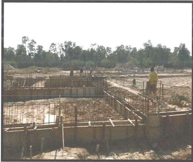
Figure 1.11 Formwork installation
