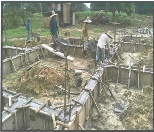
Figure 1.12 concrete work for ground beam
