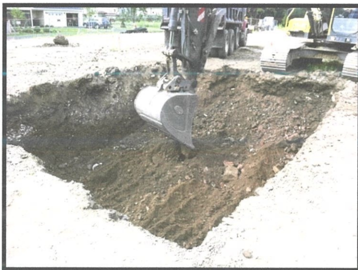
Figure 1.6 Excavations for foundation
