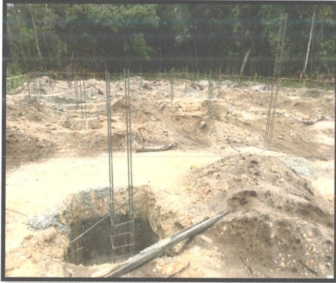
Figure 1.7 Reinforcement bar for foundation
