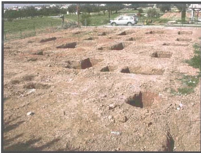
Figure 1.5 Foundation holes
