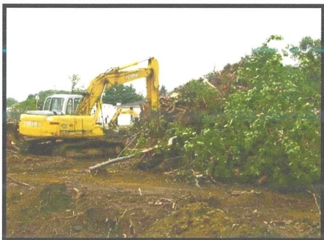
Figure 1.4 Excavator clear the tree and branches
