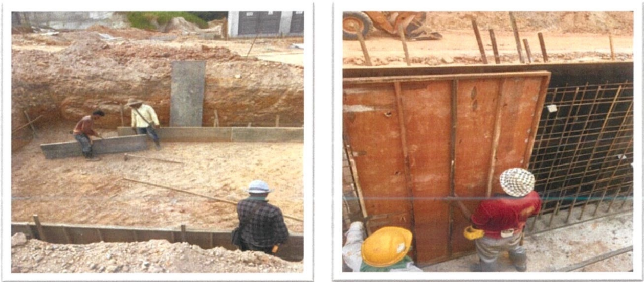
Figure 3.12 Formwork installation
