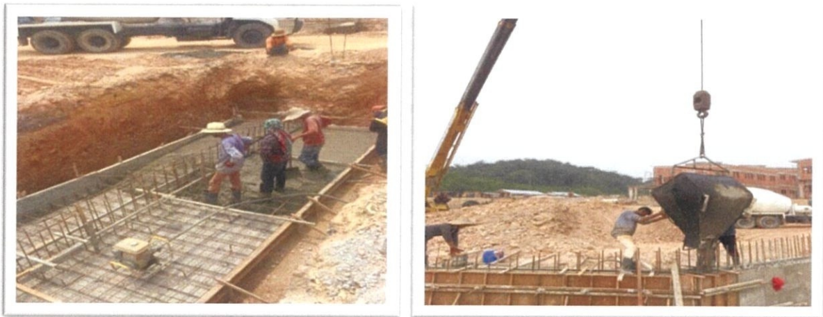
Figure 3.14: Concreting works
