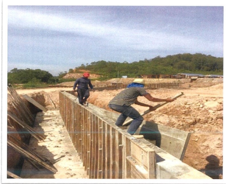
Figure 3.16 Dismantling formwork
