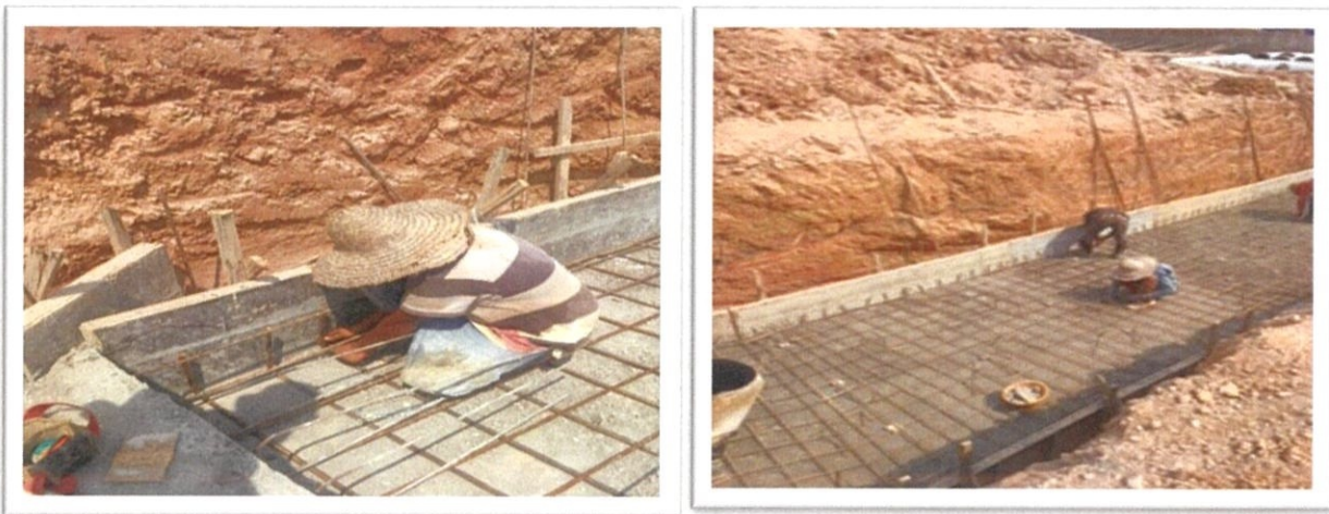
Figure 3.13: Reinforcement bar installation works for wall base
