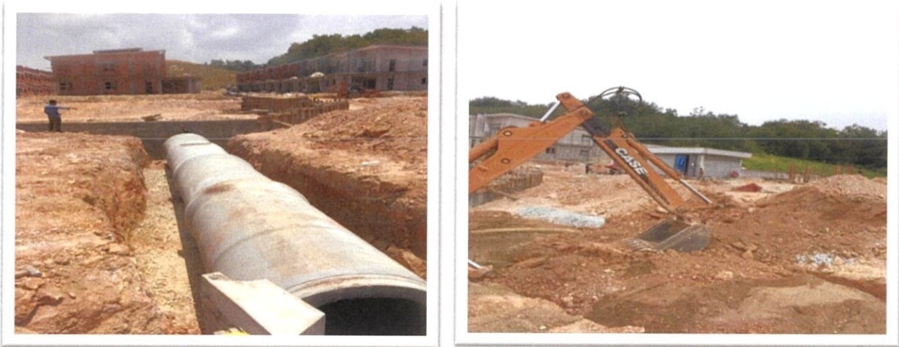
Figure 3.17: Pipe culvert installation
