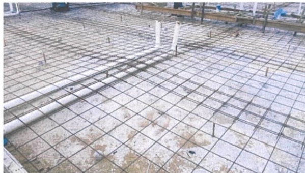
Photo 3.7: The installation of concrete floor slab
