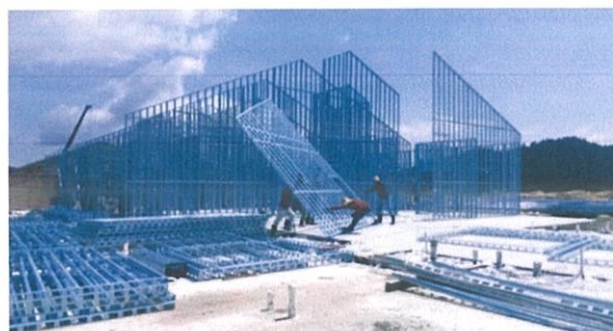
Photo 3.9: The installation of frame structures
