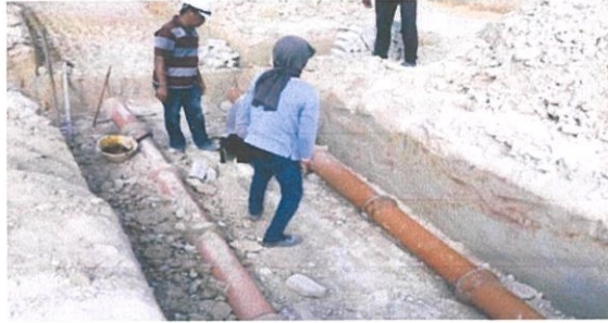
Photo 3.4: Installation of pipe
