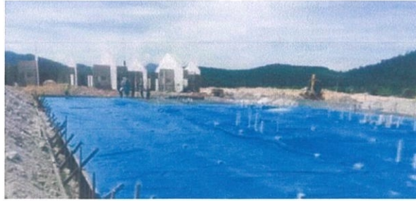
Photo 3.6: The damp proof works
