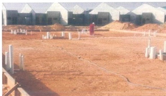
Photo 3.5: Anti-termite spray works
