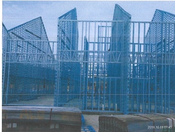
Photo 3.2 : Steel framing system
