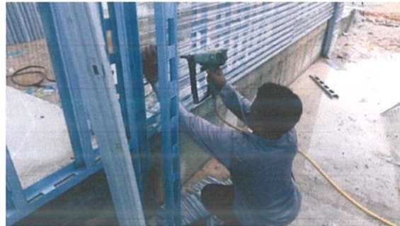
Photo 3.10: The installation of RIBLATH mesh works
