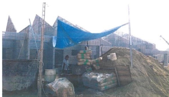
Photo 3.11: The mortar was made in the mortar filter
