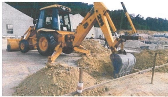
Photo 3.3: Top soil was excavated using backhoe
