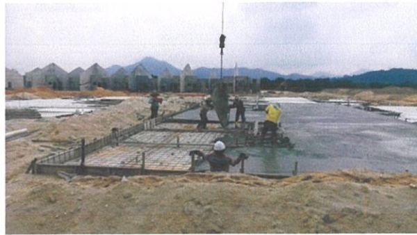
Photo 3.8: The concrete was poured by the concreters
