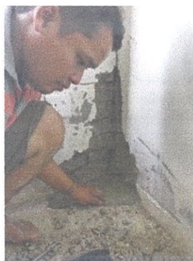
Figure 3.37: The waterproofing specialist inspecting the situation
