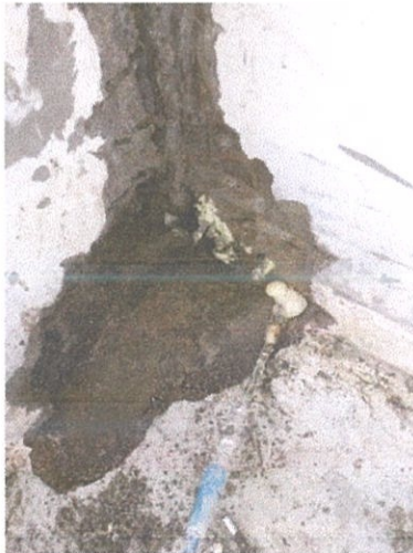
Figure 3.40: The waterproofing compound being injected
