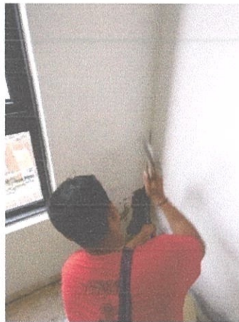
Figure 3.36: A worker hacking the wall
