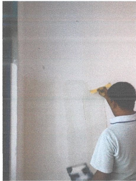
Figure 3.5: A worker applying skim coating to the wall surface
