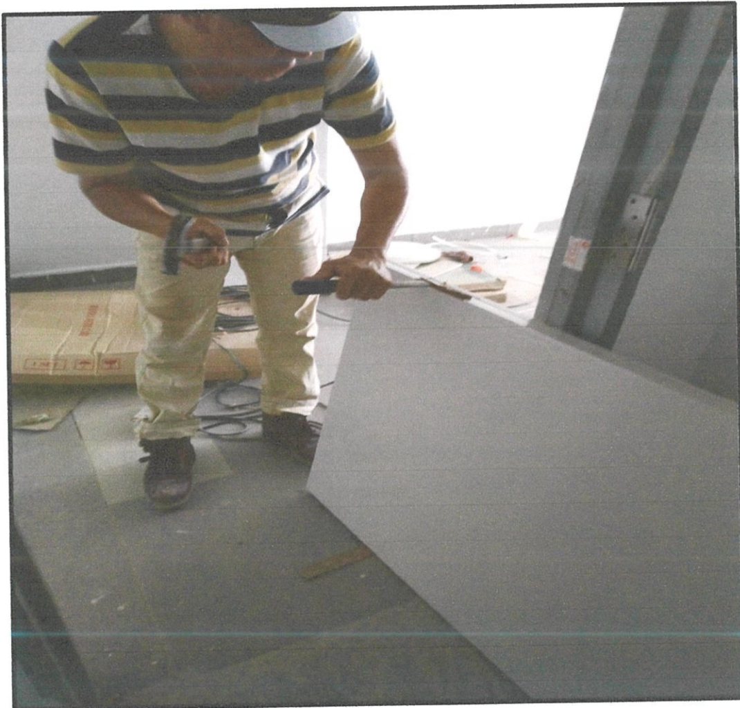
Photo 3.2: Sculpting out marked area for placing hinges
