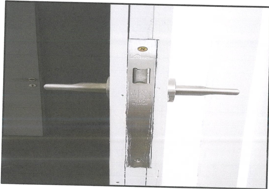
Photo 3.12 Side view of passage function lockset
