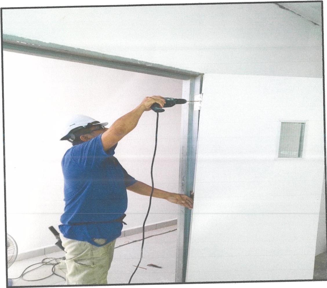
Photo 3.3 : Fix in the door leaves with screw
