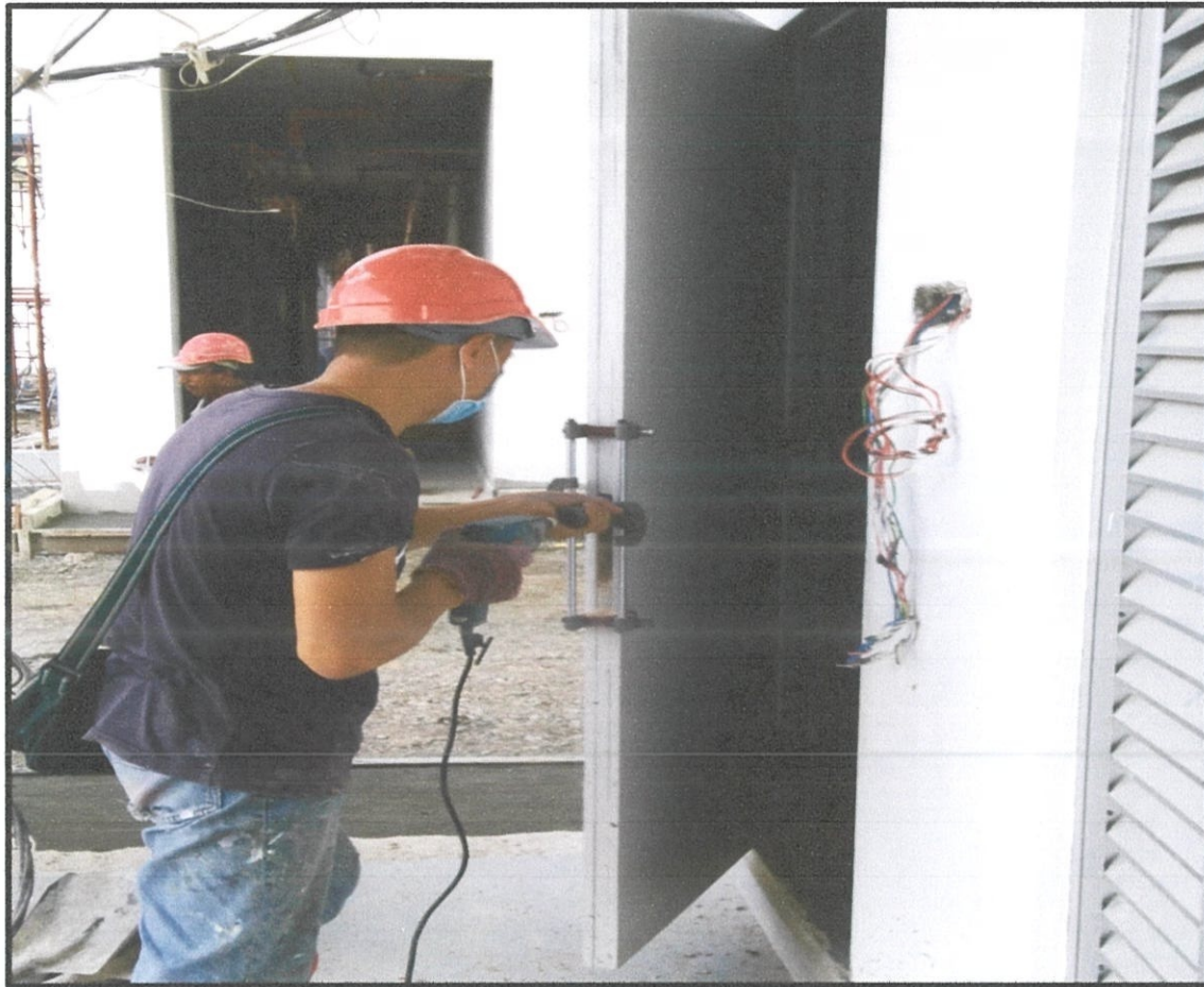
Photo 3.5 Drilling out hole for mortise lock case using special equipment
