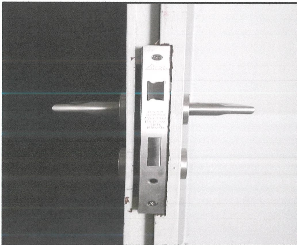
Photo 3.7 Side view of entrance function lockset
