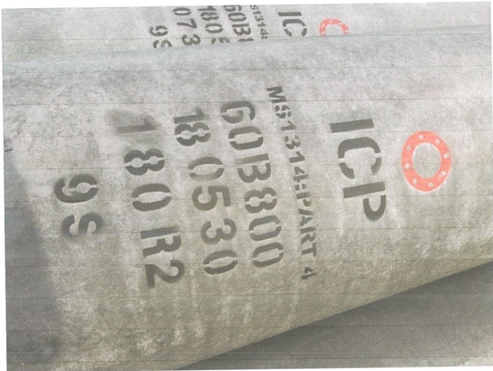
Figure 3.8 shows the specifications of spun pile
