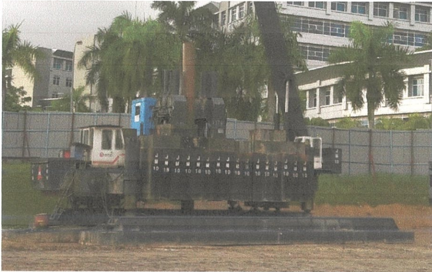
Figure 3.32 shows 2,220kN Maintained Load Test with loaded cells or block.
