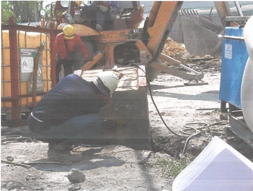
Figure 3.21 The worker prepare the hammer drop by means of welding.
