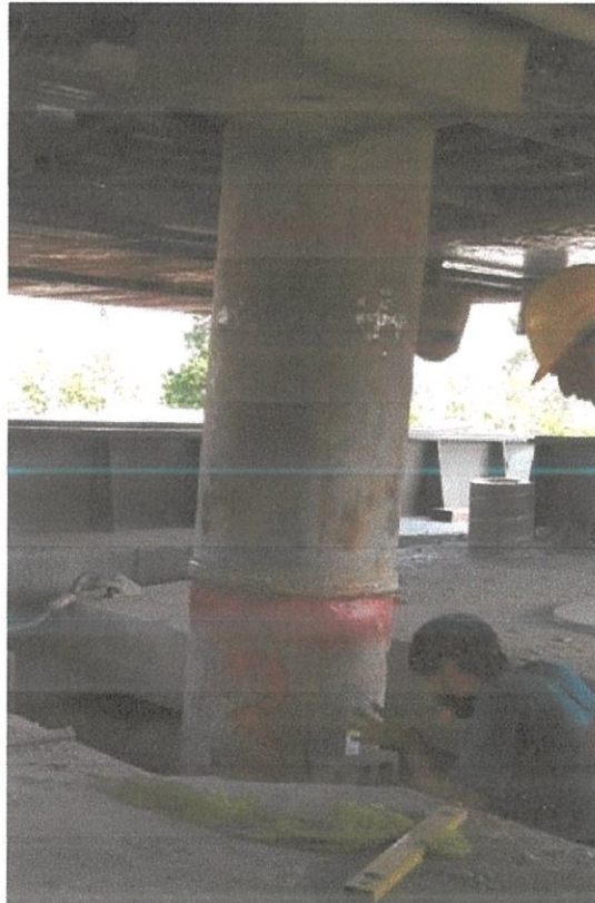
Figure 3.19 Set criteria was recorded by piling worker on graph paper.
