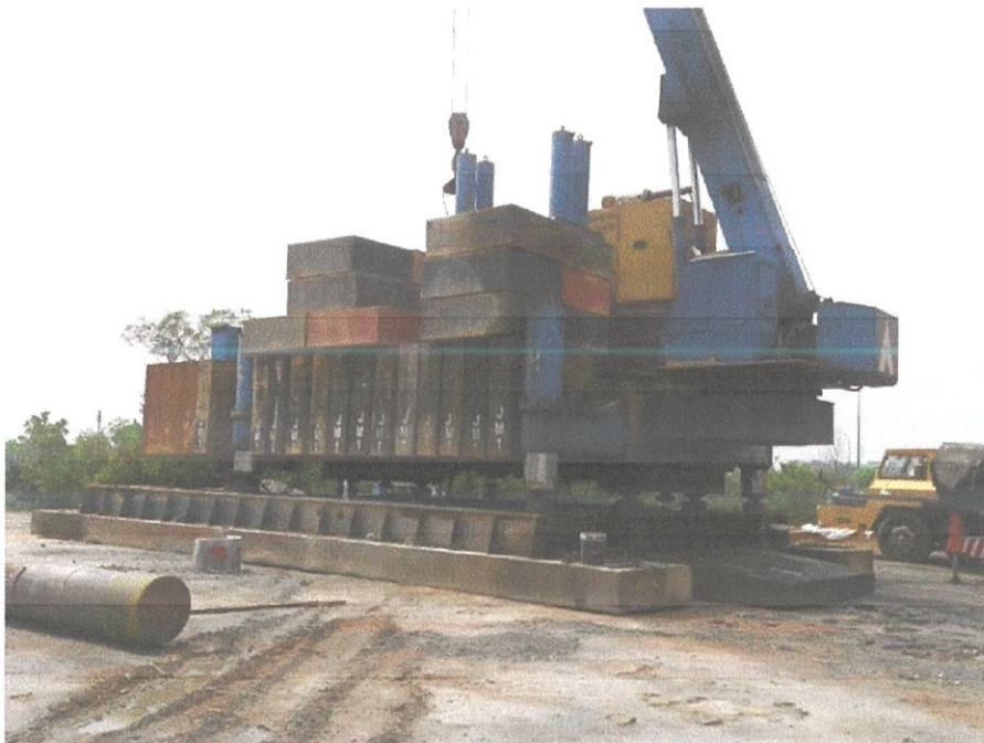
Figure 3.5 Jacked in machine
