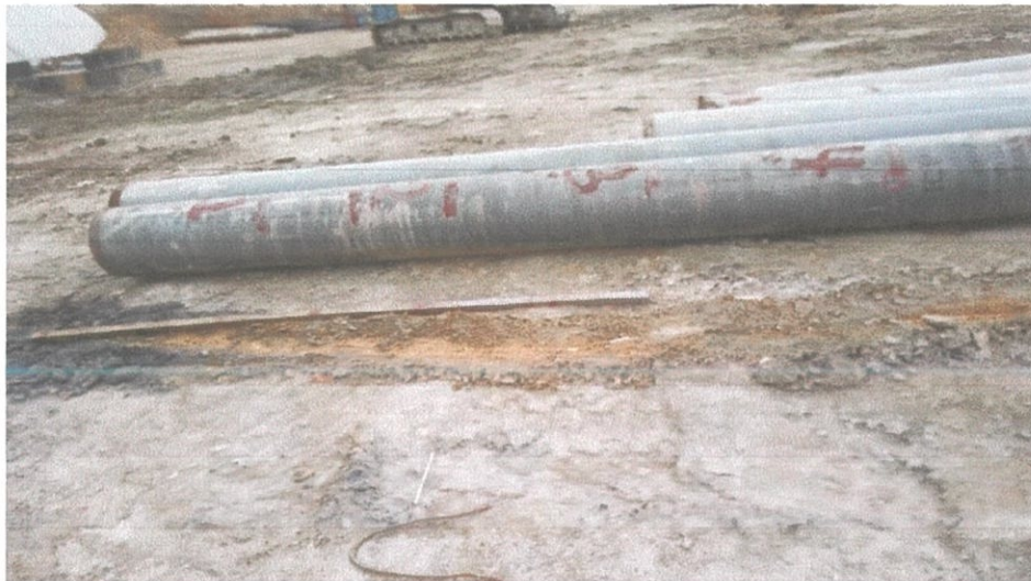
Figure 3.13 The result of painted 600mm spun pile.
