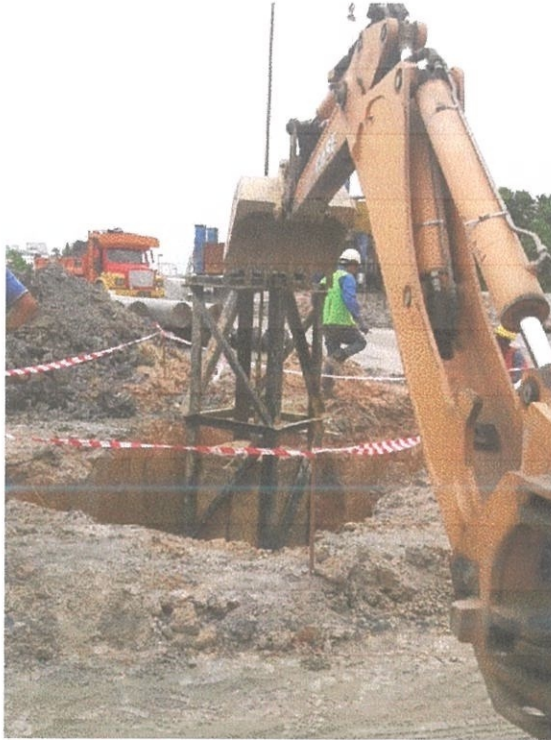
Figure 3.24 hammer drop cage secured by backhoe
