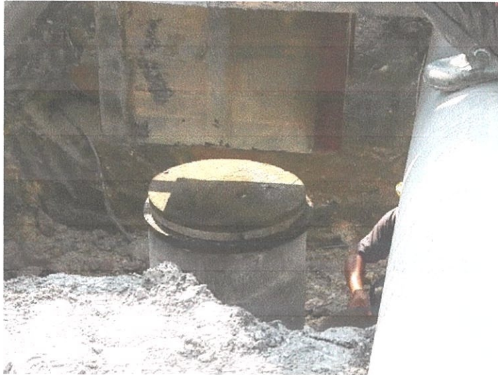
Figure 3.25 Tested pile need to be covered by timber cushion.
