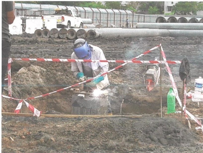
Figure 3.29 SLT workers prepared welding equipment on tested pile
