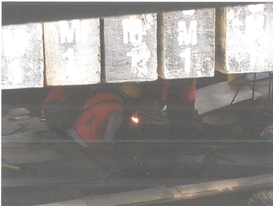
Figure 3.16 Welding process of extended 600mm spun pile
