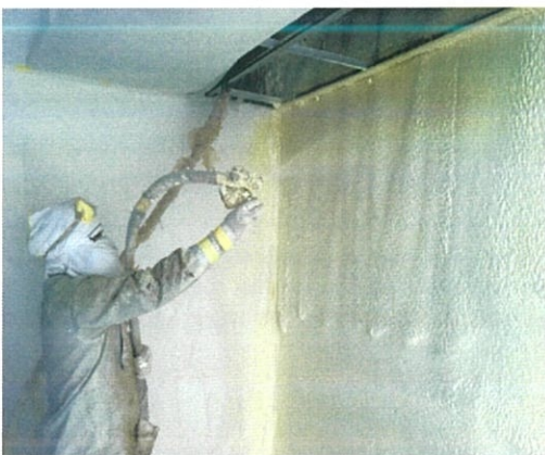
Figure 3.42: SPF in progress
