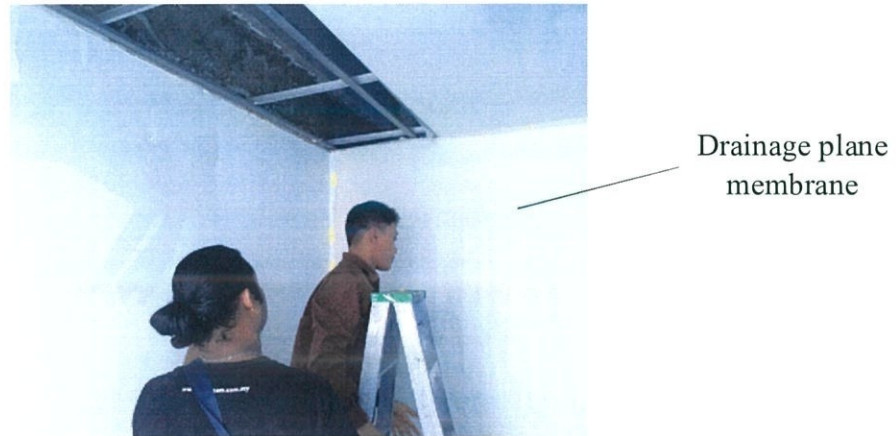
Figure 3.41: Drainage plane membrane
