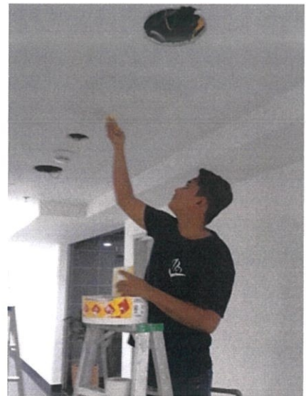
Figure 3.16: Worker install first skim coat layer
