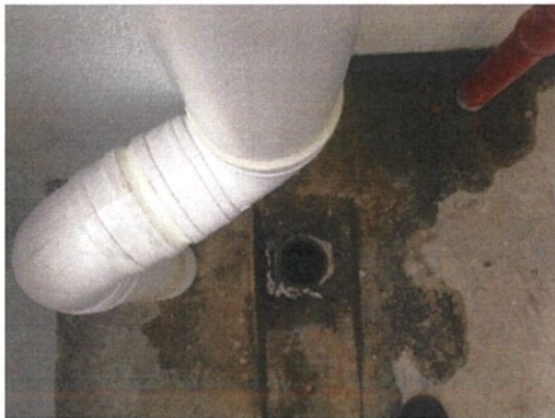
Figure 1.3: Clogged Trap
