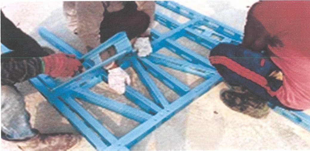
Photo 3.18: Steel was joined together
