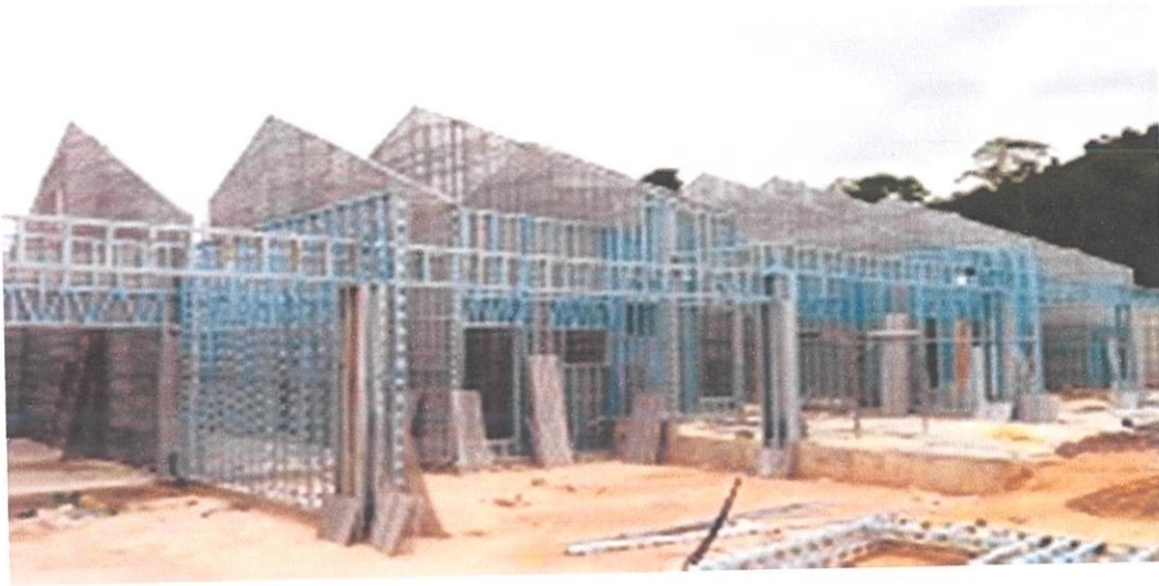
Photo 3.16 : Wall panel Type B
