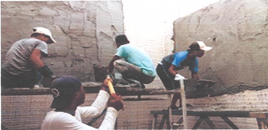
Photo 3.26: plastering work
