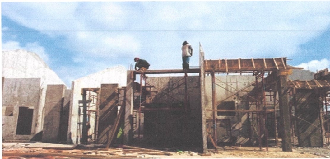
Photo 3.15: formwork
