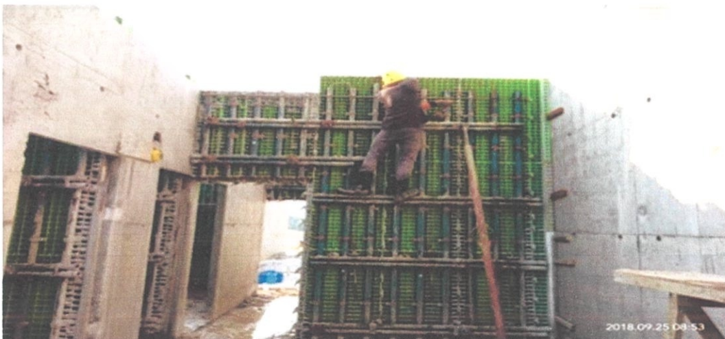
Photo3.7: Mould for wall panel
