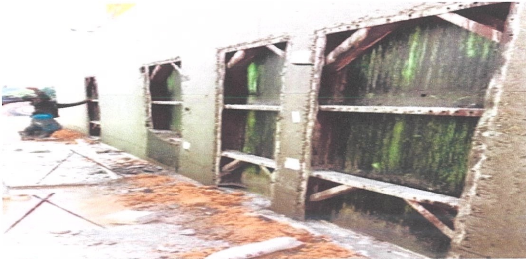
Photo3.14: Inside the mould
