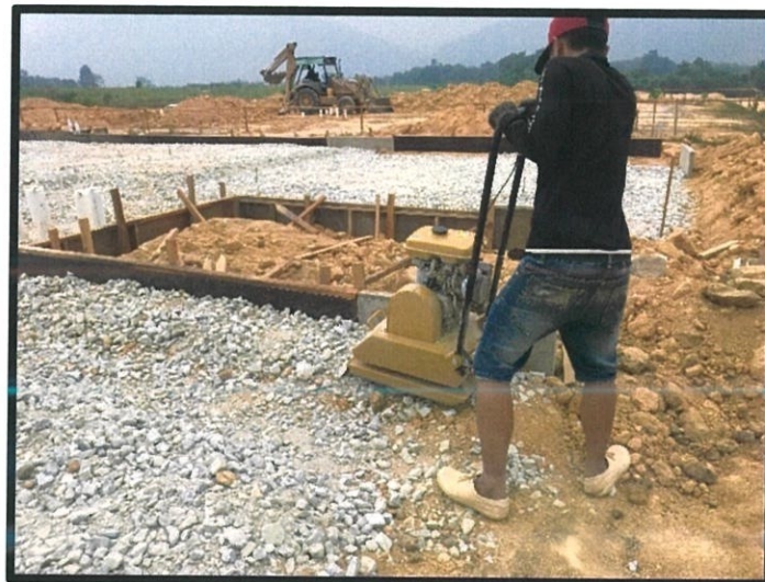
Figure 3.15 Workers compact the crusher run
