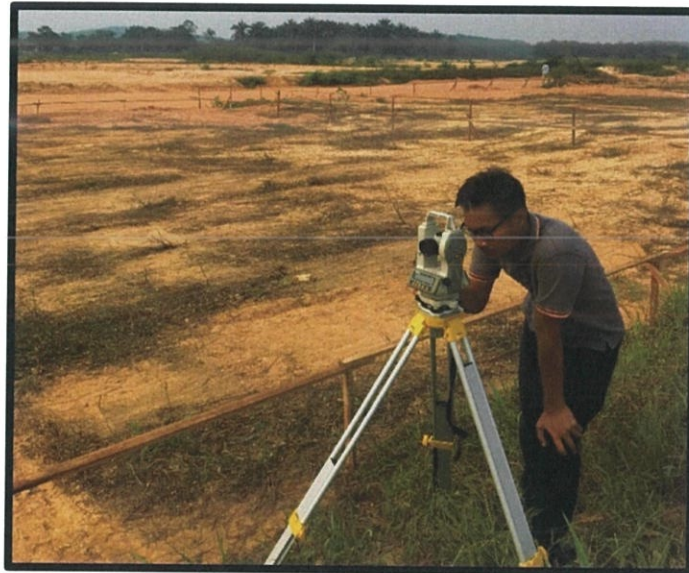
Figure 3.3 Setting out work
