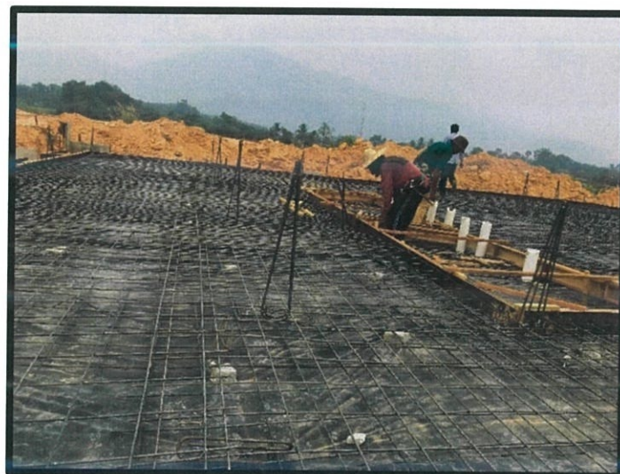
Figure 3.23 Reinforcement bar for raft foundation
