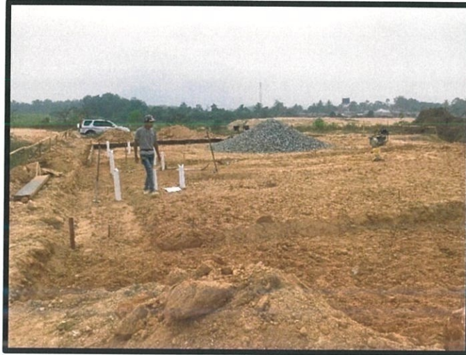
Figure 3.10 Excavate 150mm thickness
