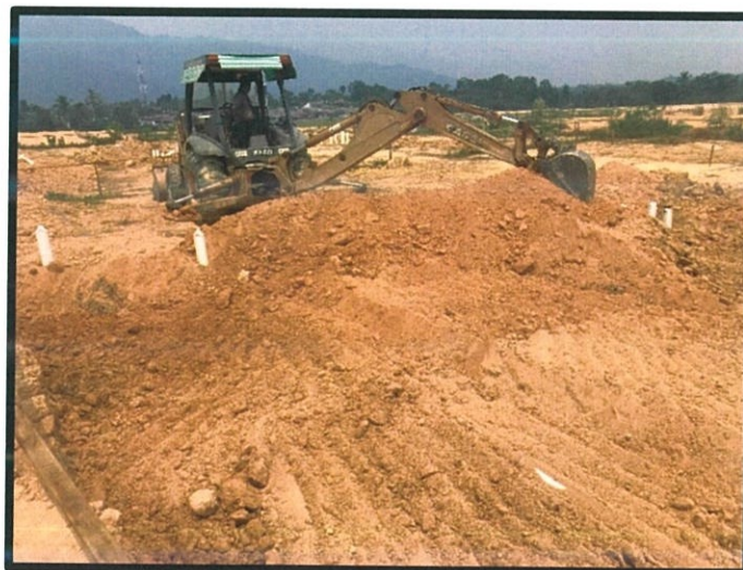
Figure 3.9 Backhoe excavate top soil
