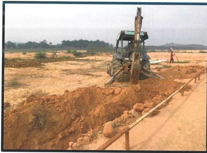
Figure 3.6 Backhoe digging trench
