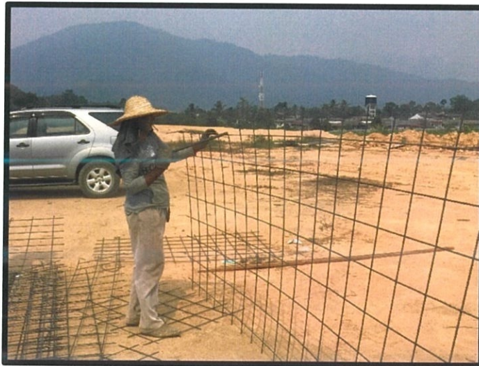
Figure 3.21 The worker preparing BRC A7 for slab
