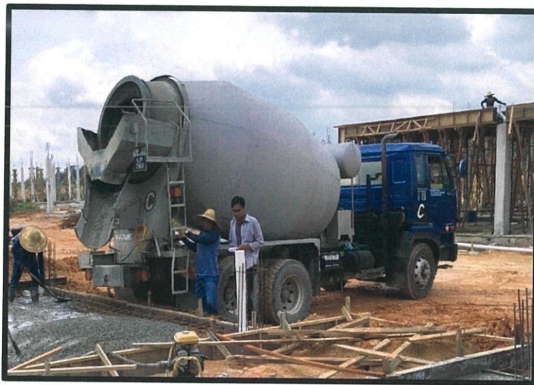
Figure 3.30 The concrete mixer
