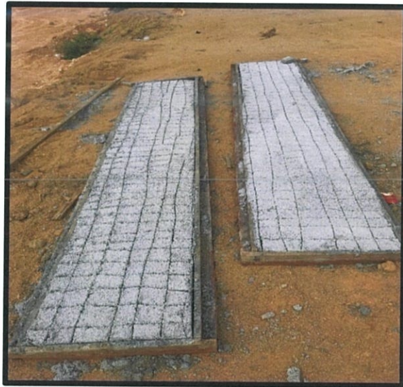
Figure 3.24 Preparing spacer block
