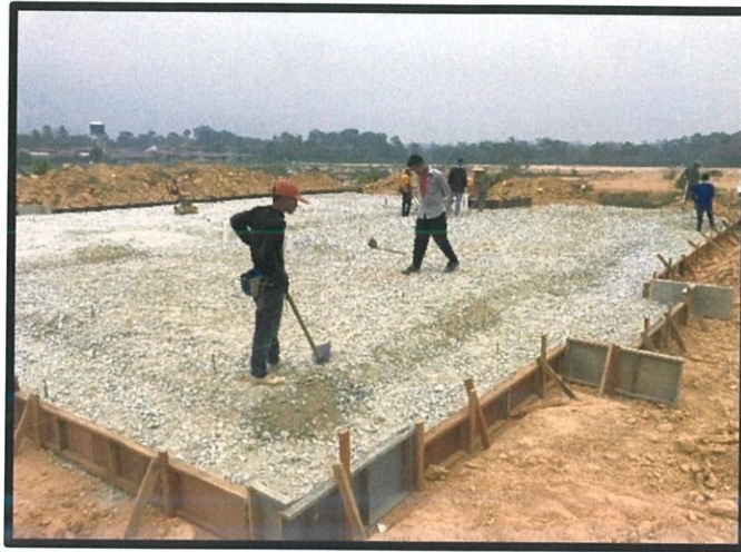
Figure 3.14 The workers level the crusher run
