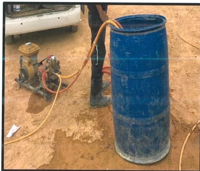
Figure 3.17 Using water jet to spread the anti-termite
