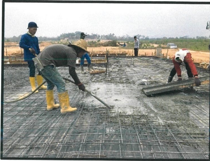
Figure 3.28 Workers compact the concrete using vibrator
