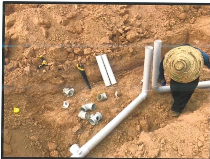
Figure 3.7 Plumber install the pipe
