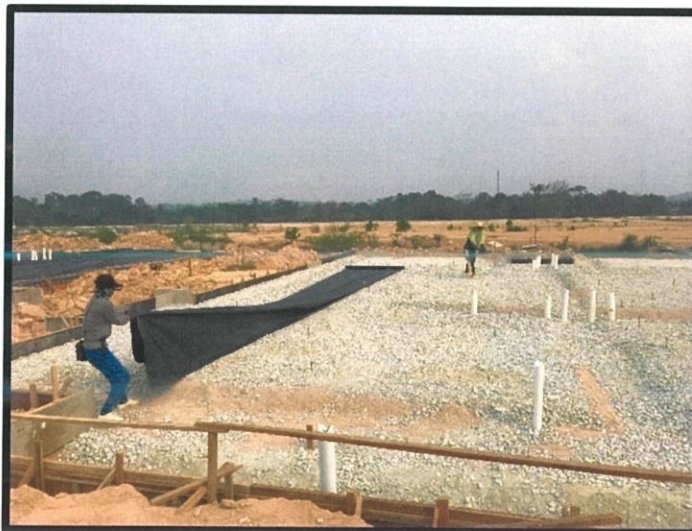
Figure 3.19 Workers laying polythene sheet
