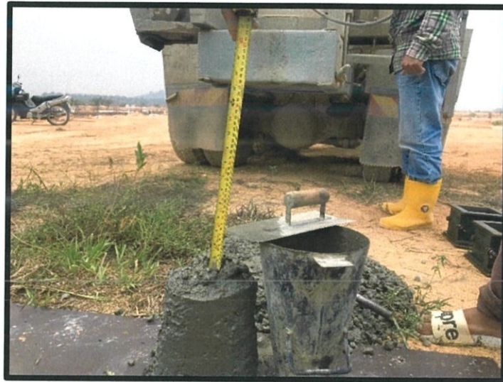
Figure 3.26 Slump test 75 mm and cube on site
