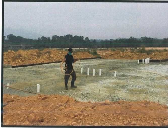
Figure 3.18 Worker spread the anti-termite
