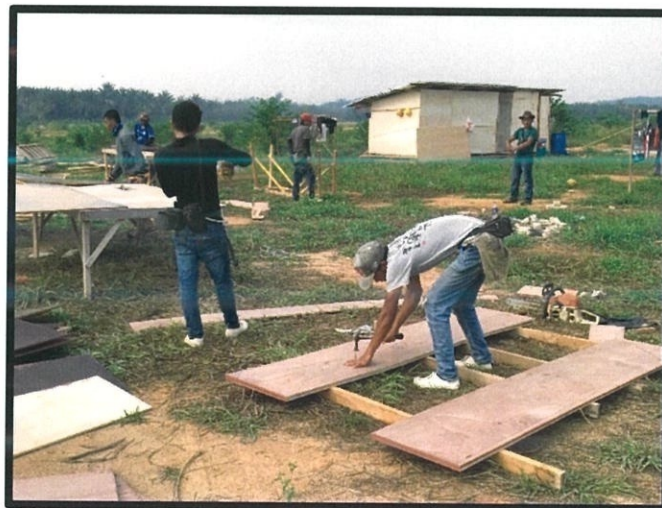
Figure 3.11 Workers preparing formwork
