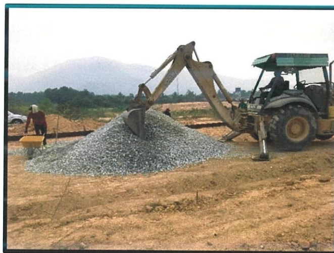
Figure 3.13 The backhoe spread the crusher run
