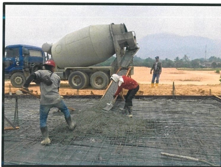
Figure 3.27 The workers spread the concrete
