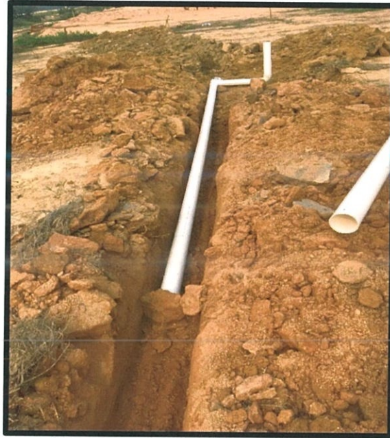
Figure 3.8 Backfill the trench
