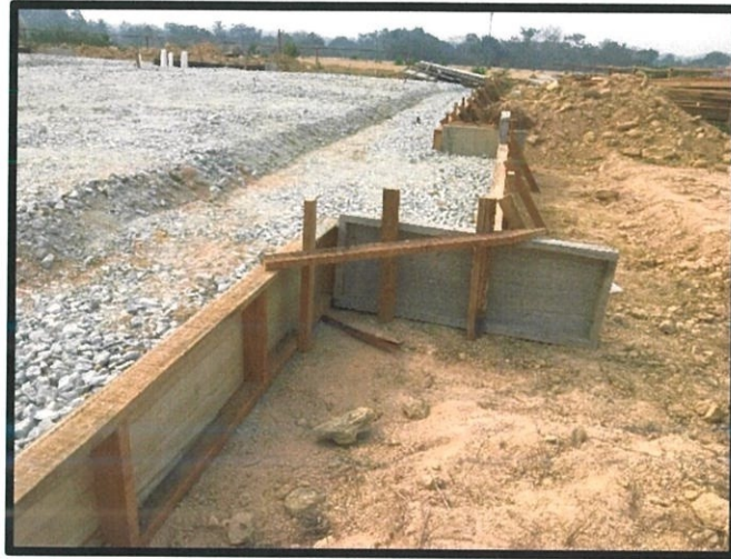
Figure 3.12 Install formwork at raft foundation
