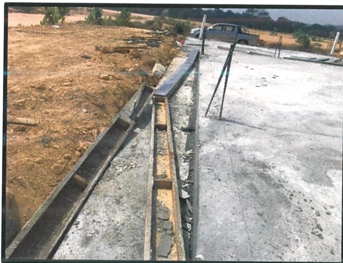
Figure 3.29 Dismantle the formwork of raft foundation
