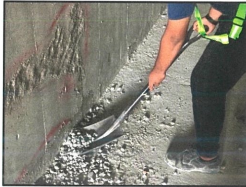
Figure 10: Clear debris and dust
