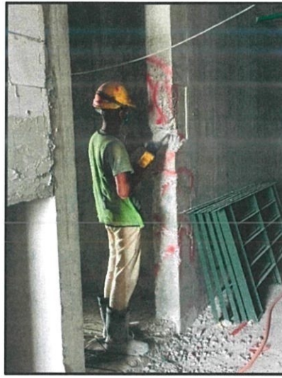
Figure 8: Hacking work
