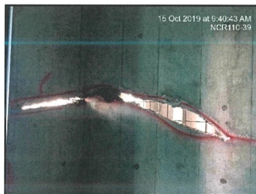
Figure 9: Hacking surface that reach firm surface
