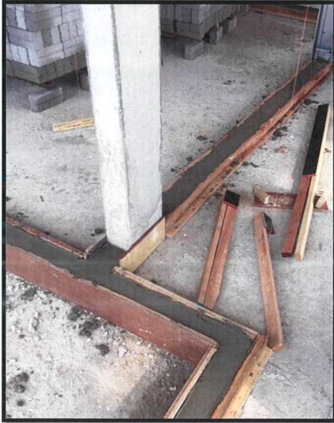
Figure 3.6 Kicker at ground slab.
