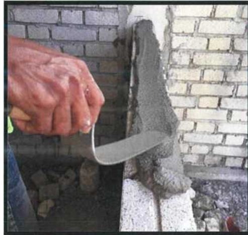
Figure 3.11 Mortar spreading by using a trowel.
