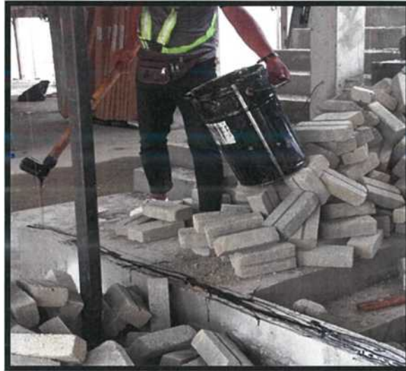
Figure 3.7 Hot bitumen application.
