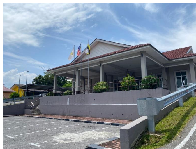
The MAIPk Tapah's office building
