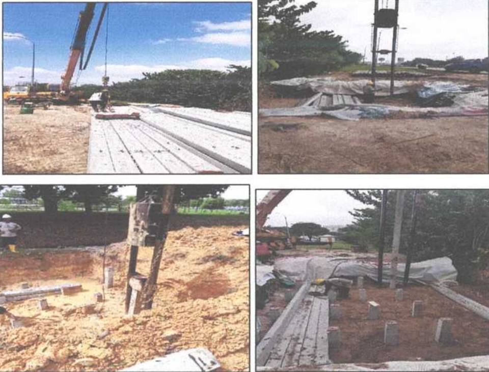
Figure 5.0: Piling Works (Courtesy of FE Sdn Bhd)
