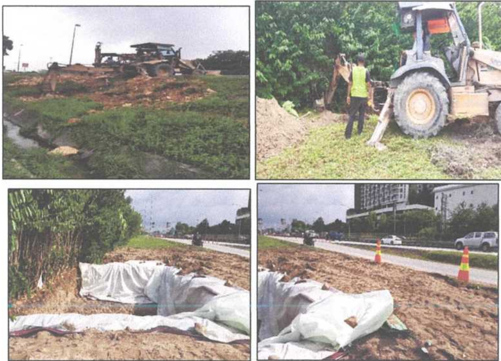
Figure 4.0: Excavation Works (Courtesy of FE Sdn Bhd)
