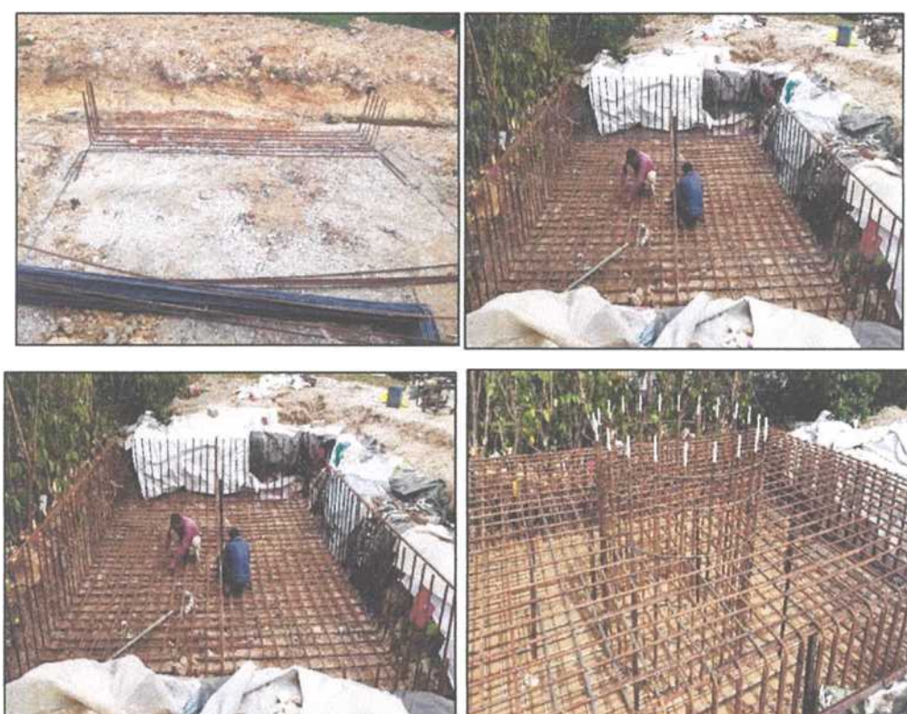
Figure 6.0: Installation of Reinforcement Bar (Courtesy of FE Sdn Bhd)
