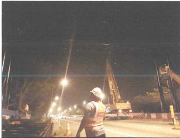
Figure 9.0: Launching Works (Courtesy FE Sdn Bhd)
