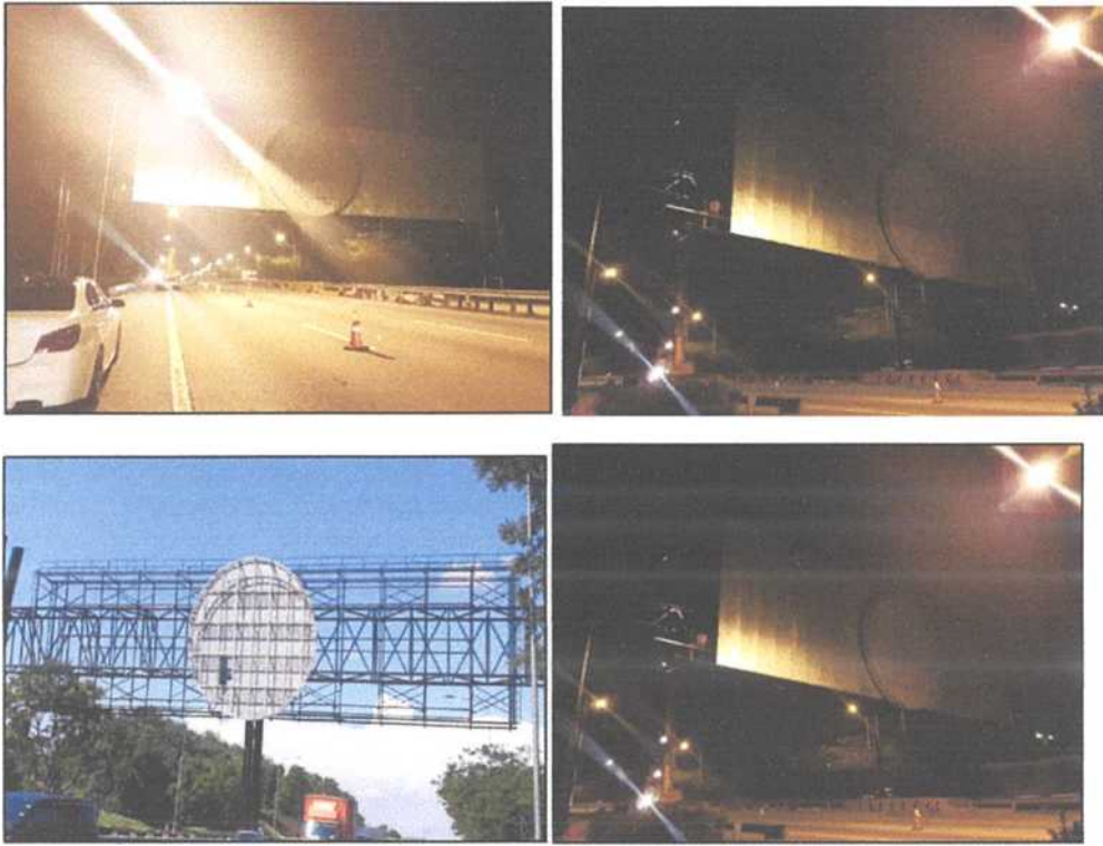
Figure 10.0: Installation of Ads Panel (Courtesy FE Sdn Bhd)
