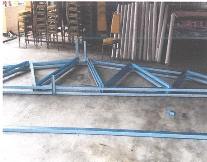
Figure 3.6 Truss before erected
