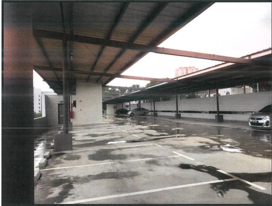
Figure 3.8 : Parking garage at Level 7, MKH Boulevard
