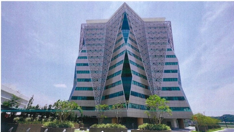
Figure 3.1.5: Completed construction of Block F11
