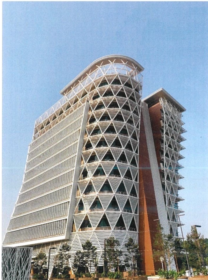
Figure 3.1.3: Completed construction of Block F05
