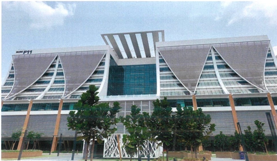
Figure 3.1.4: Completed construction of Block F11
