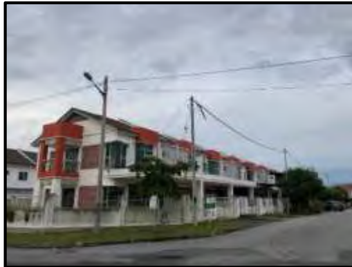
Figure 2: Residential Building at Seri Iskandar
