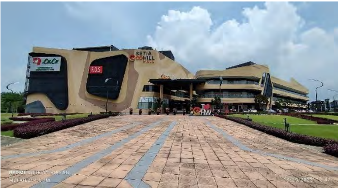
Figure 1: Front View Setia Ecohill Mall
