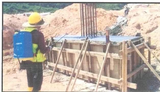
Figure 3.2.11(a): Spraying curing compound to pile cap
