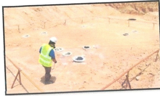
Figure 3.2.6(a): Spraying curing compound
