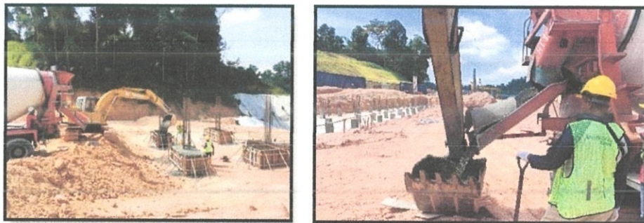
Figure 3.2.10(a): Concreting work for pile cap
