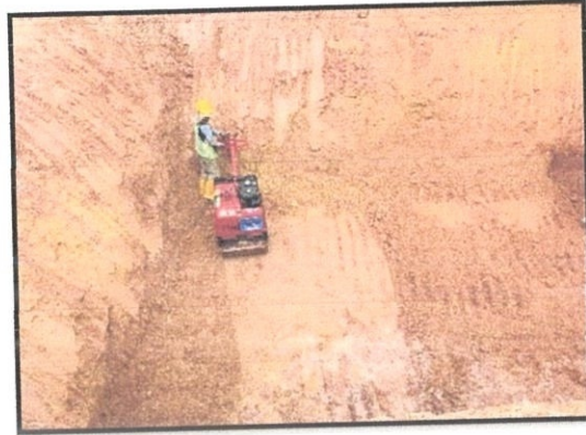
Figure 3.2.4(a): Compaction of soil
