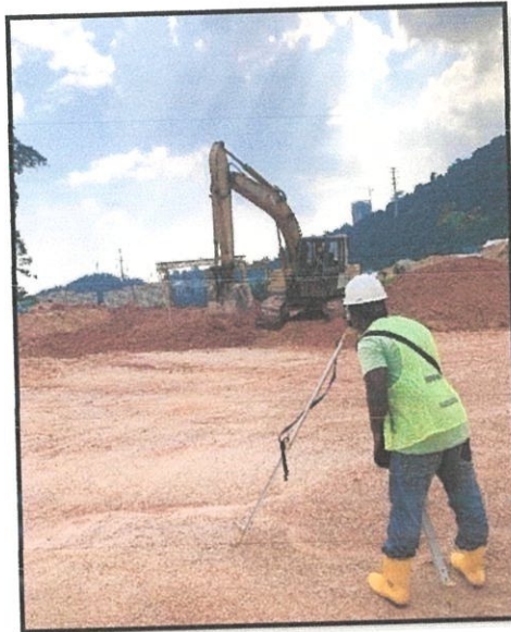
Figure 3.2.2(a): Surveying work
