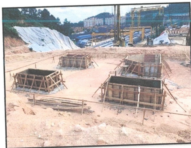
Figure 3.2.8(b): Formwork of pile cap
