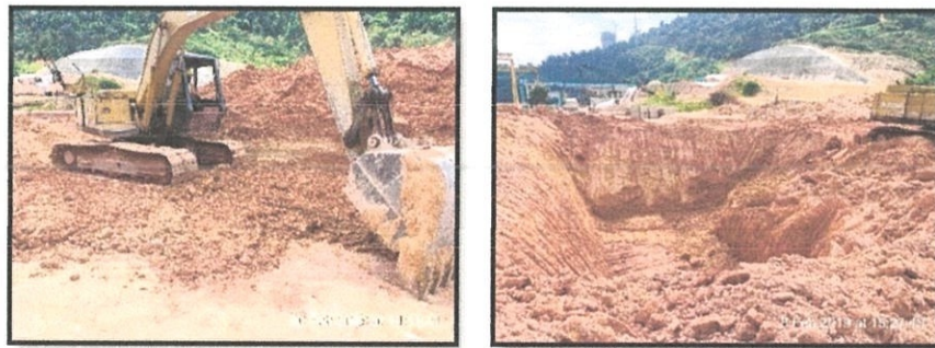
Figure 3.2.1(a): Excavation work on site
