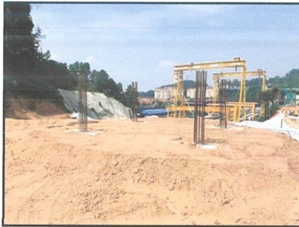
Figure 3.2.13(a): Pile caps Backfilled
