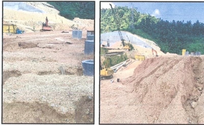
Figure 3.3(a): Sedimentation of soil
