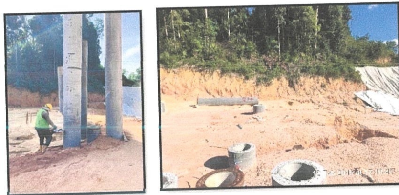
Figure 3.2.5(a): Cutting of spun piles
