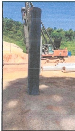
Figure 3.2.2(c): Drive of addition pile
