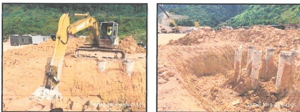
Figure 3.2.3(a): Excavation work for pile caps
