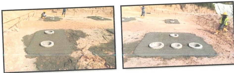
Figure 3.2.7(a): Lean Concrete for Pile Caps
