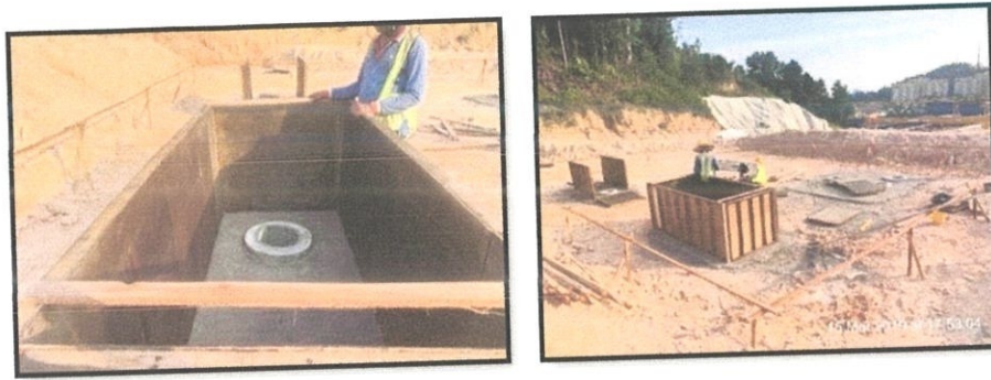
Figure 3.2.8(a): Process of erecting of formwork for pile caps
