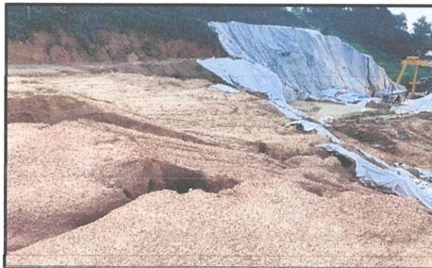
Figure 3.3(b): Geotextile laid to slopes
