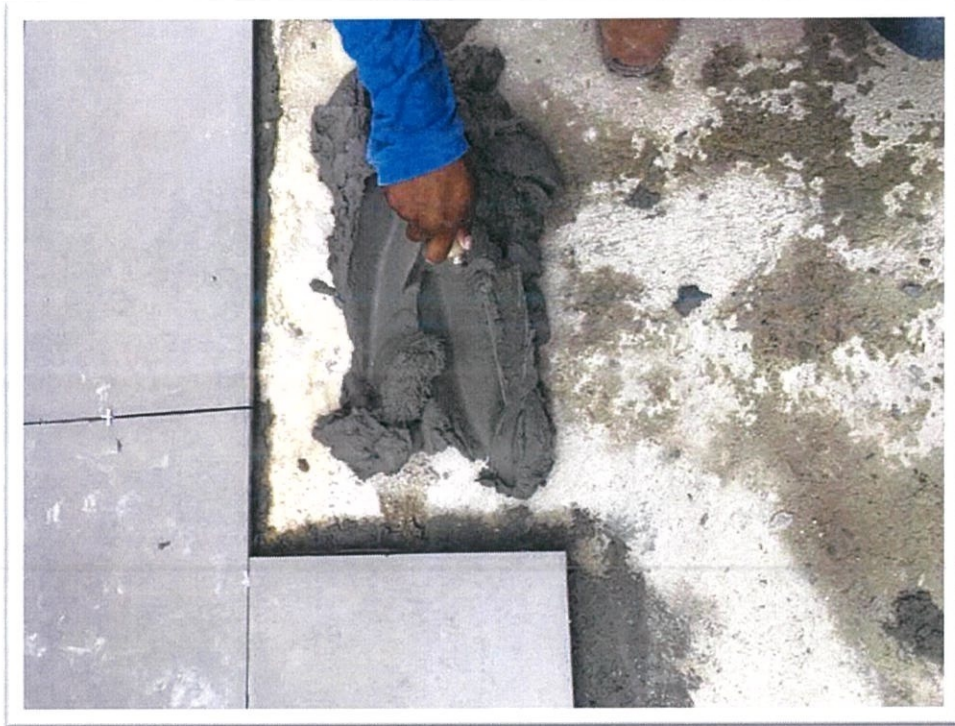
Figure 3.7: Apply Adhesive
