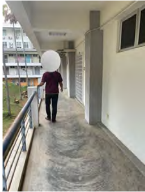
Figure 5: Respondent walking at the corridor while holding the handrail
