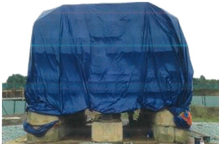
Figure 1.3 Side view of Static Load test (Kentledge)
