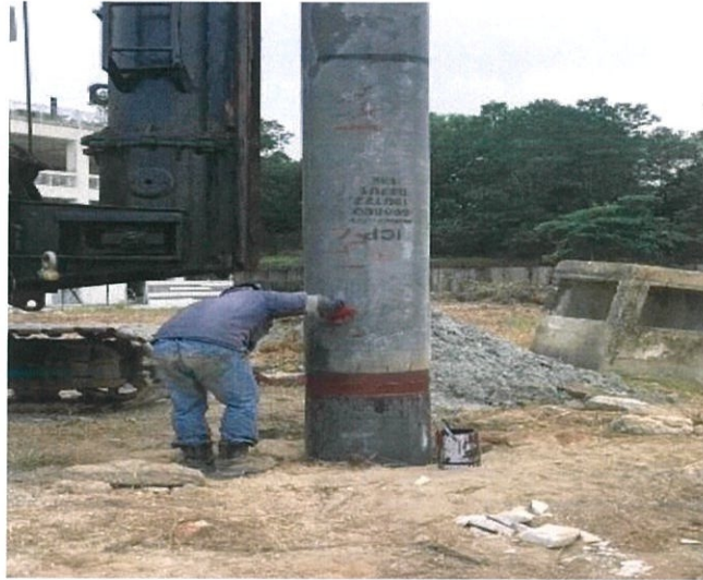
Figure 3.11: Pile installation at point number 374
