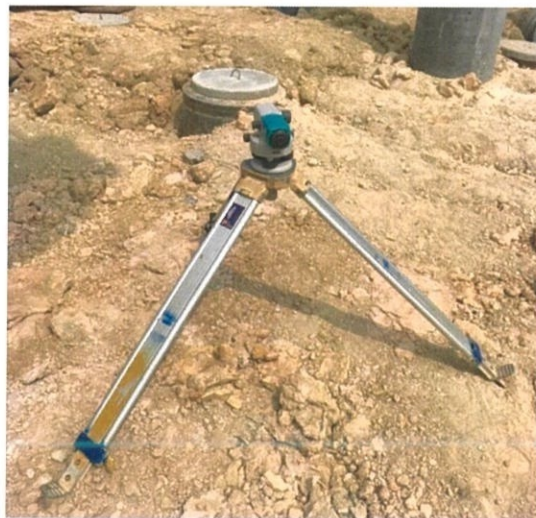
Figure 3.24: Dumpy Level is succcefully set up
