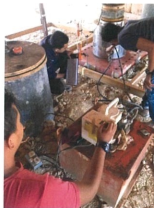
Figure 3.21: Hand Pump is connected by hose to hydraulic jack
