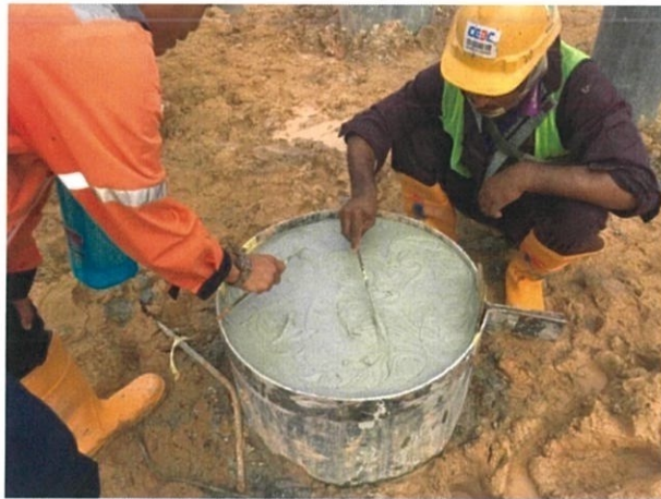
Figure 3.12: Nitomortar is added to harden the pile surface
