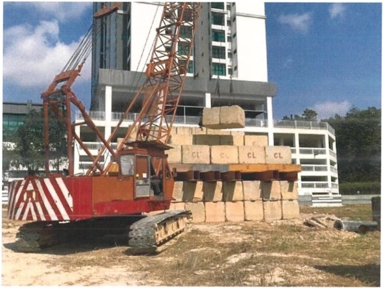
Figure 3.13: Block arrangement using crawler crane
