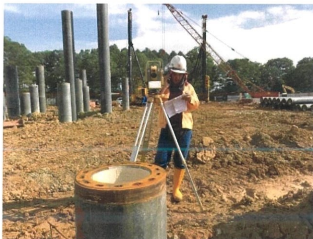
Figure 3.6: Setting out pile point using Total Station
