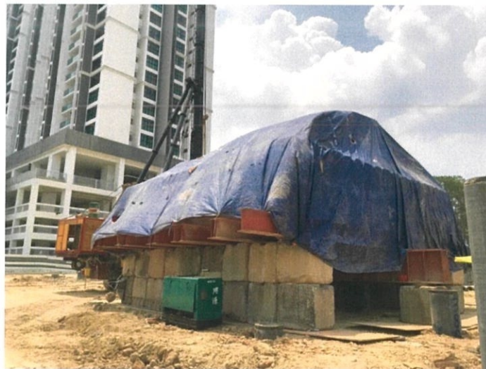
Figure 3.26: Overall look of Maintain Load Test from outside
