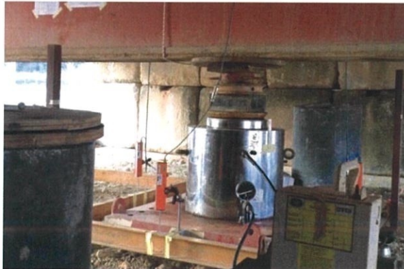
Figure 3.18: Hydraulic jack with steel bearing plate
