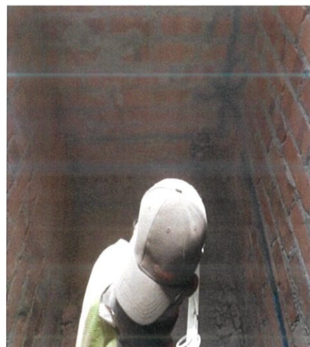
Figure 6.1 Brick wall cutting for hacking work
