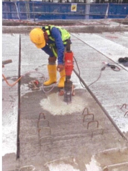
Figure 4.4 Coring the slab using the coring machine
