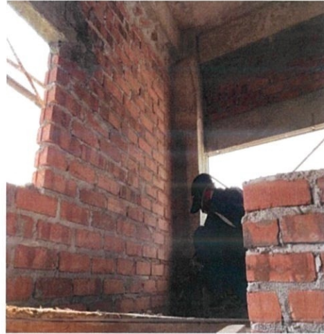
Figure 6.3 Hacking work for conceal
