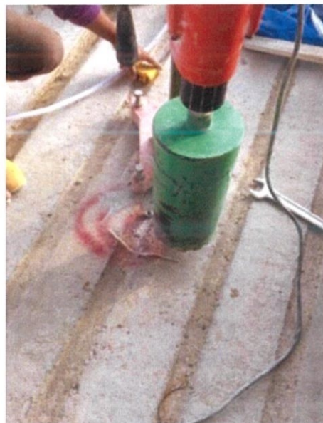
Figure 4.3 Adjust and centralized the coring machine
