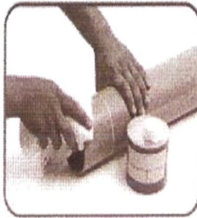
Figure 5.2 Cleaning process (source: Tetuan Yeo Plumber Sdn Bhd)
