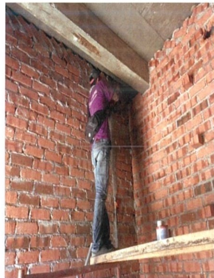
Figure 5.6 The installation of Upvc pipe at high level
