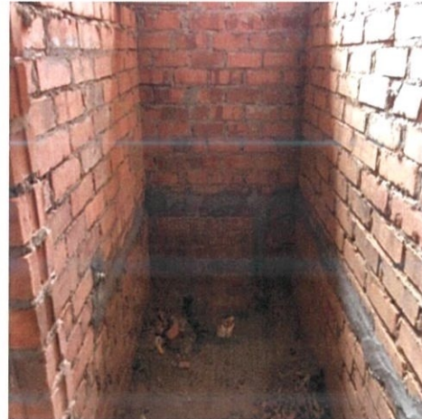
Figure 6.5 Installation of cement mortar
