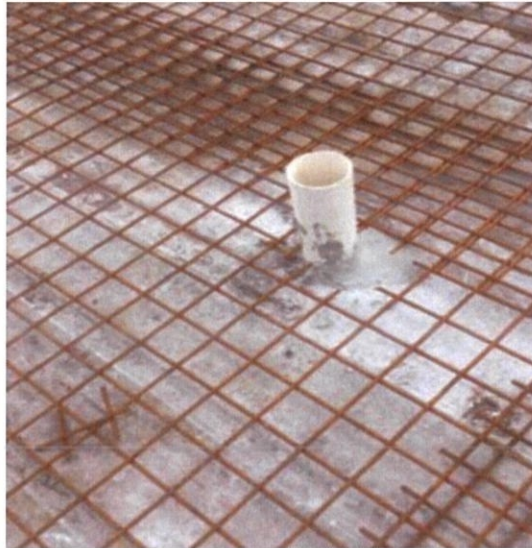
Figure 4.6 Upvc pipe installation at rooftop
