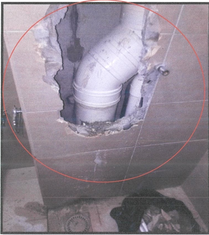
Photo 3. 10: Rainwater downpipe inside box up area
