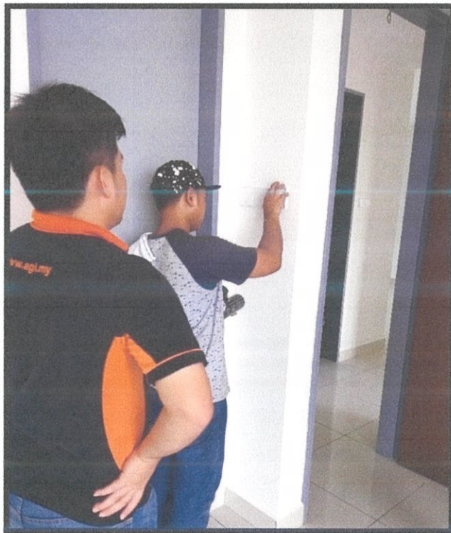
Photo 3. 6: Inspection with the clerk work
