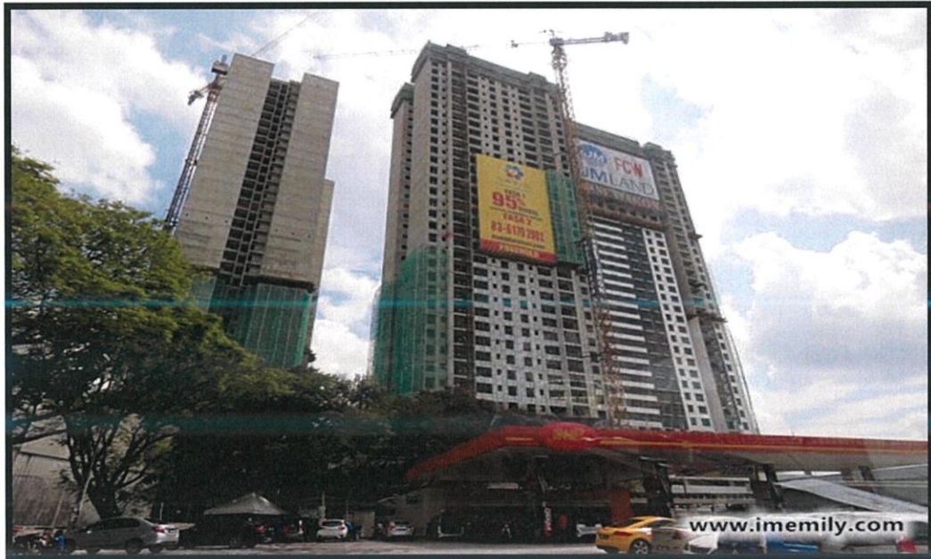
Figure 3.2 : Riana Dutamas's site from beside of the road
