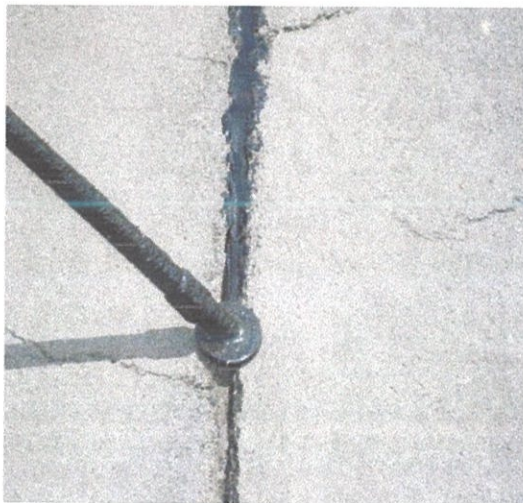
Figure 28 Filled the crevice with filler
