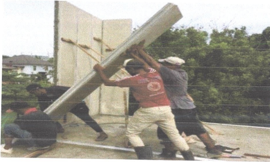
Figure 9 Installing panel wall.
