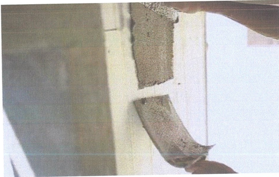
Figure 17 Skim coating the jointing.
