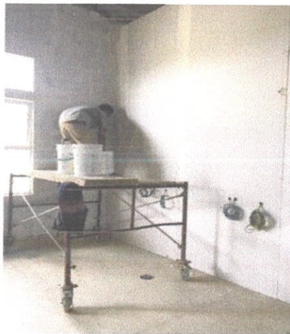
Figure 26 Applying Skim Coat
