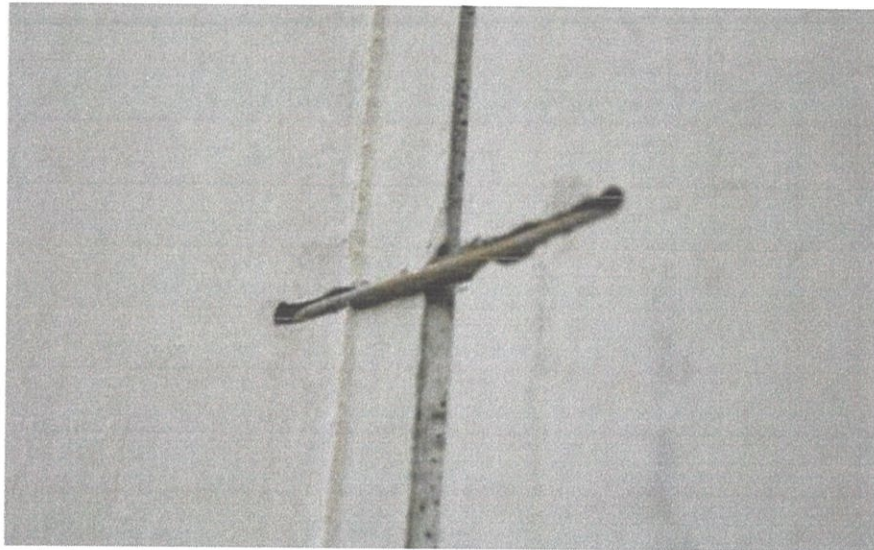
Figure 15 Stapling each panel.
