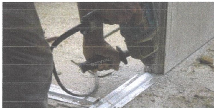
Figure 12 Drilling the bottom track.
