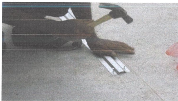
Figure 7 Nailing the bottom track.
