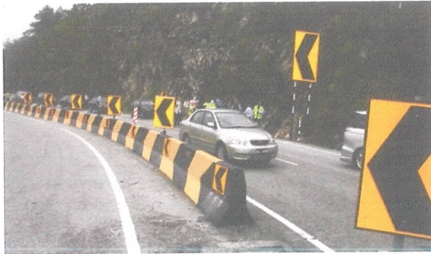
Figure 3.4: New Jersey Barrier
