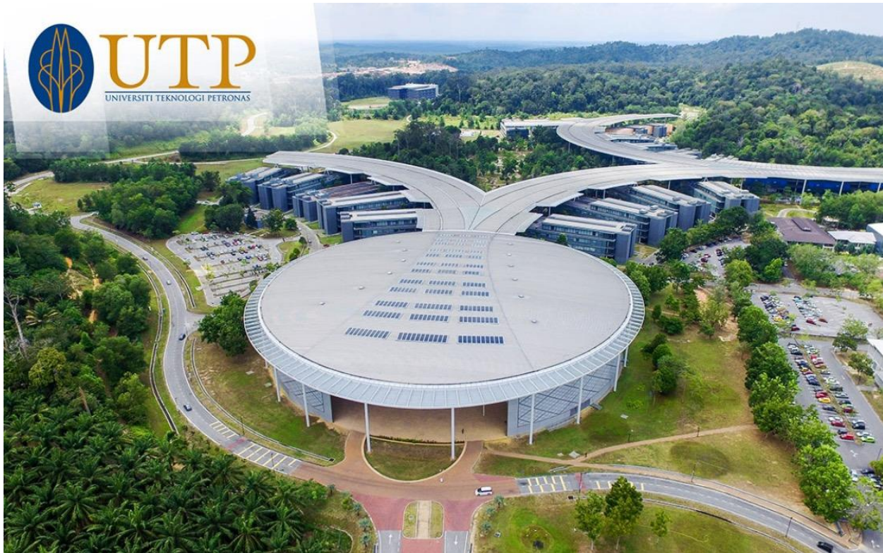
Figure 3.2: Overview of the building
