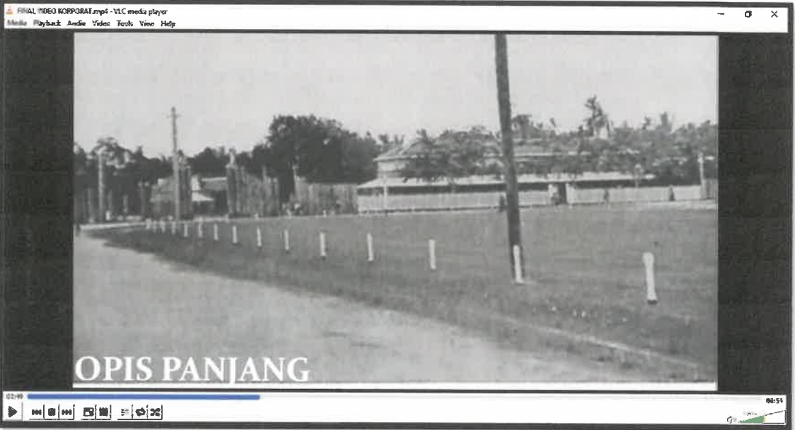
Figure 29: Old building of Kelantan state secretary office
