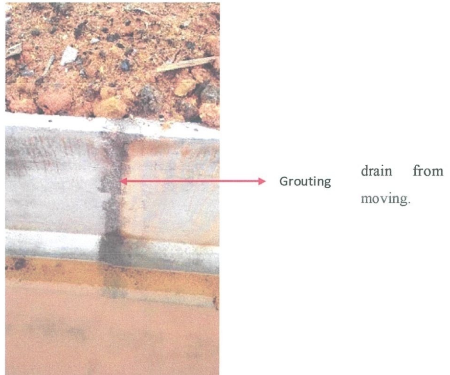
Figure 3.9 show the grouting between the precast U-drainage.
