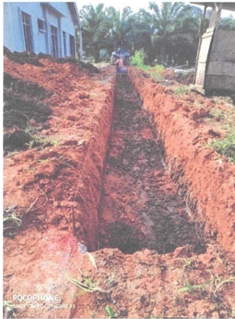
Figure 3.10 show the does not have any gravel during installation process.
