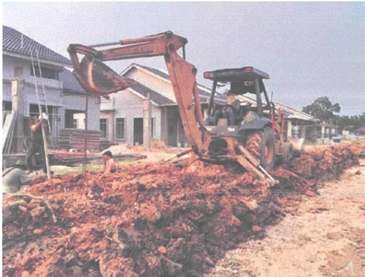
Figure 3.5 show the backhoe is digging
