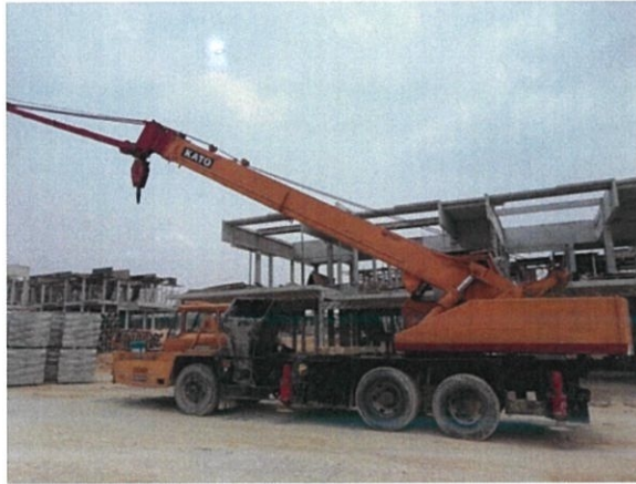
Figure 3.22: Crane on site.
