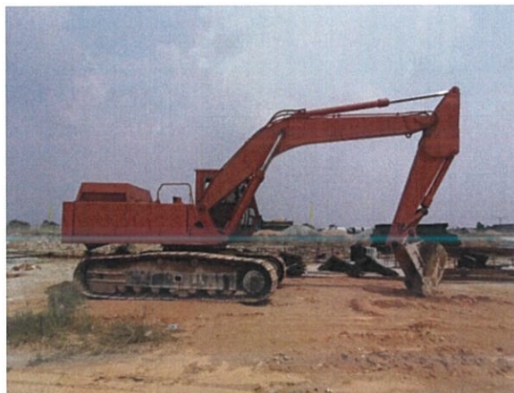
Figure 3.23: Excavator on site.
