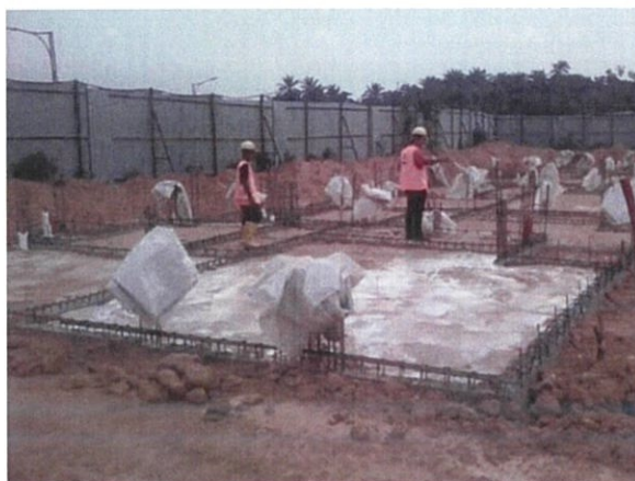
Figure 3.6: Application of anti-termite on soil.
