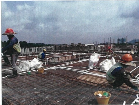
Figure 3.12: Installation of M&E works.
