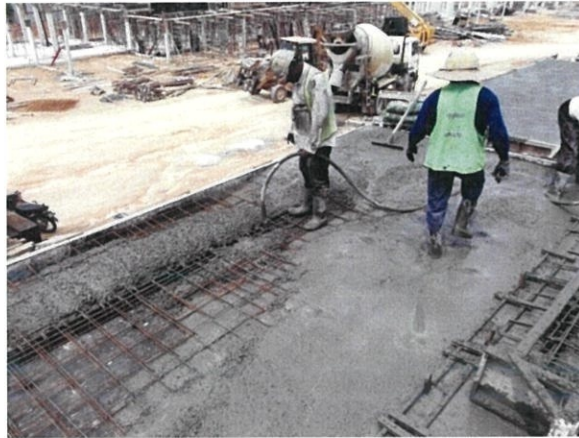
Figure 3.17: Concreting work which vibrator was used to compact the concrete.
