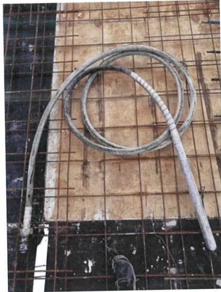
Figure 3.24: Vibrator poker to compact concrete.
