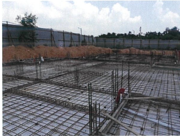
Figure 3.8: Installation of reinforcement bars at ground slab.
