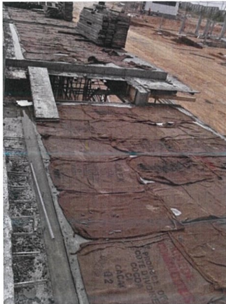
Figure 3.18: Wet hessian cloth was used for curing process.
