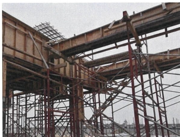
Figure 3.7: Installation of formwork and supports at roof beam and slab.
