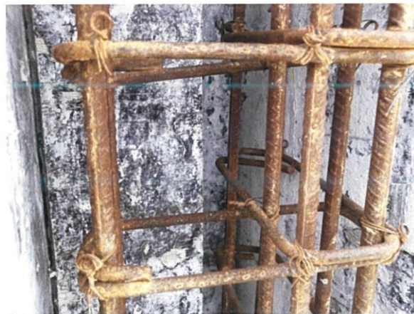
Figure 3.9: Fixation of links at column.
