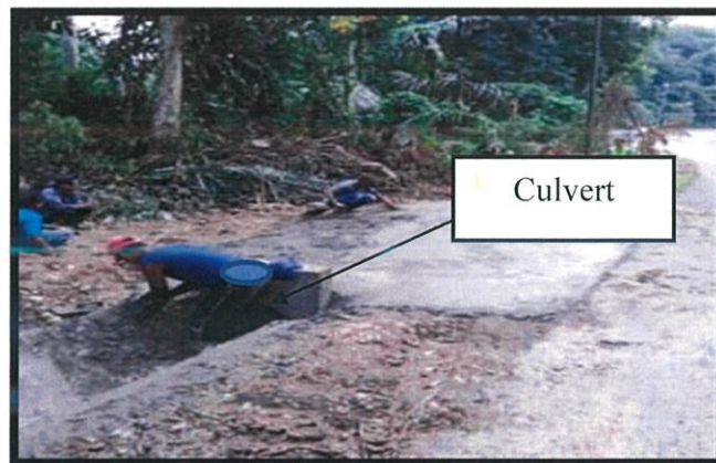
Photo 3.19: Work outside the culvert is carried out.
