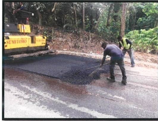
Photo 3.13: Hand casting works
