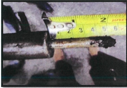
Photo 3.15: Premix thickness measured
