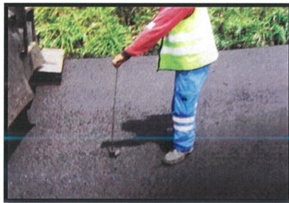
Photo 3.14: Dipping to check premix thickness
