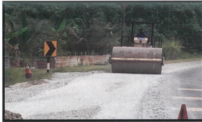
Photo 3.5: Compaction of crusher run
