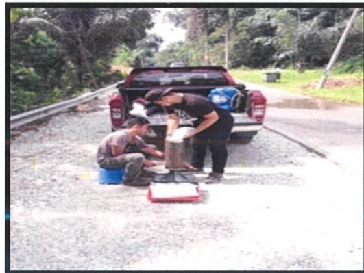
Photo 3.8: Sand is filled into the cone
