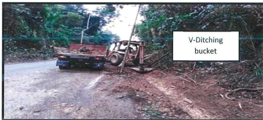
Photo 3.22: Roadside drain excavation.
