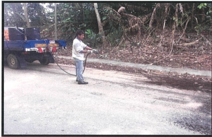
Photo 3.9: Tack Coat is sprayed
