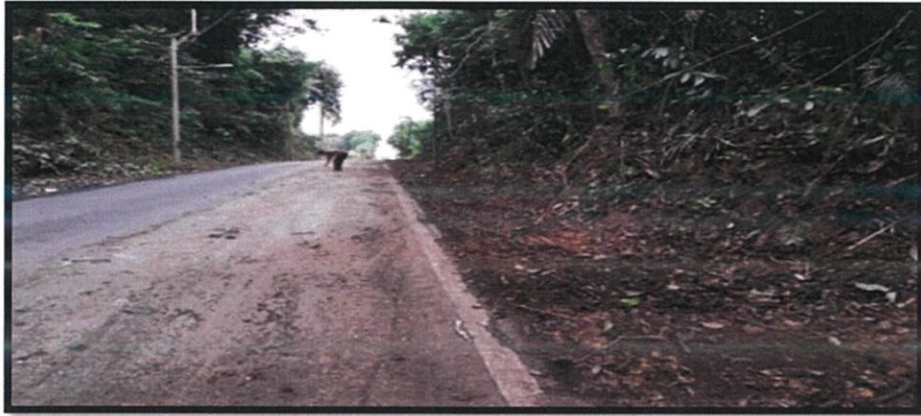
Photo 3.21: Roadside cleaning work for roadside drain.
