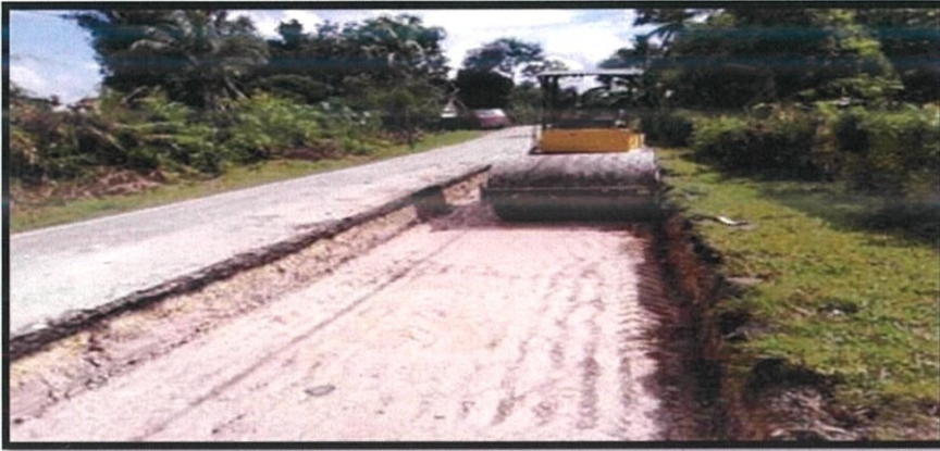
Photo 3.4: Sand compacted with roller machine
