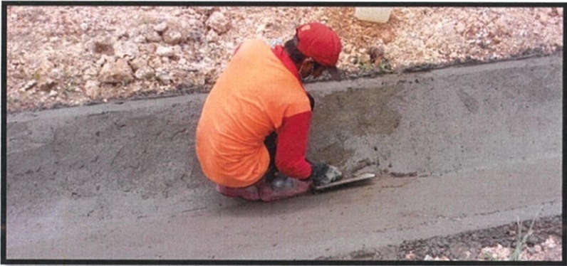
Photo 3.24: Cement screed by workers.
