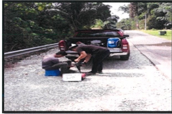
Photo 3.7: Excavated crusher run for field density test
