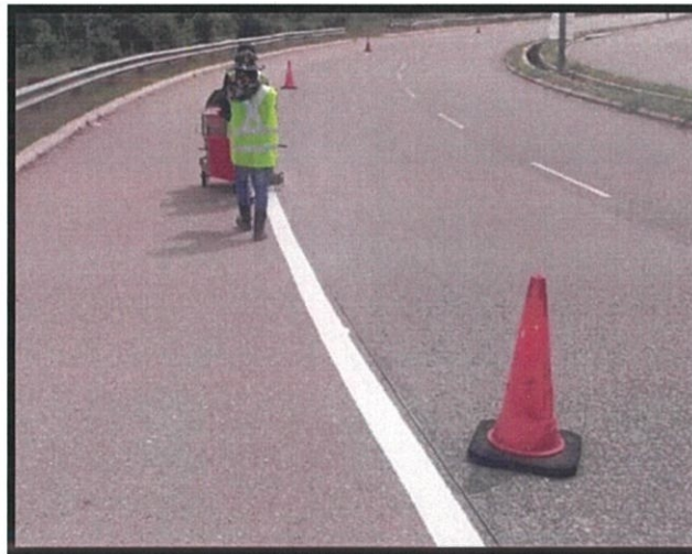
Figure 3.2: Road marking in progress
