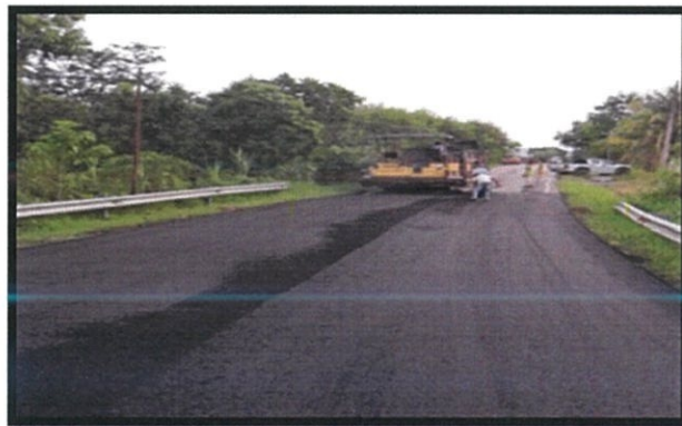
Photo 3.10: Road pavement in progress.
