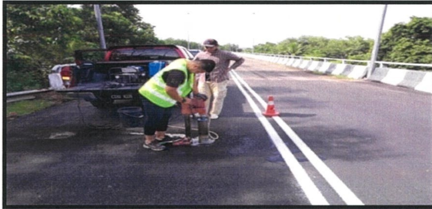
Photo 3.17: Coring test performed by the workers
