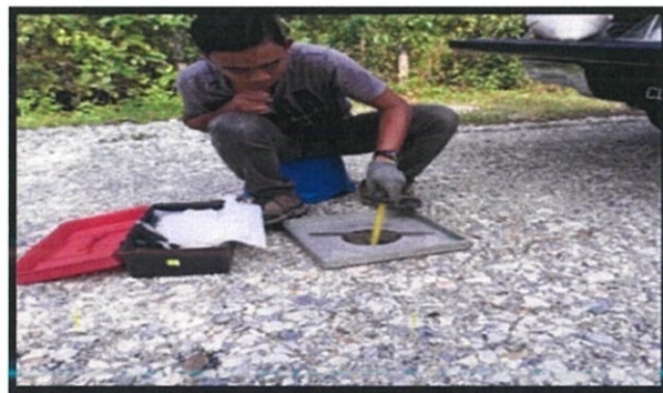
Photo 3.6: Worker check excavated depth
