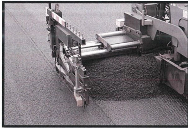
Figure 3: Paver screed control
