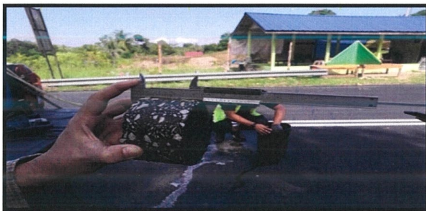
Photo 3.18: Pavement thickness depth check.
