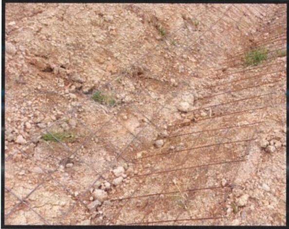
Photo 3.23: Square mesh applied on both side.
