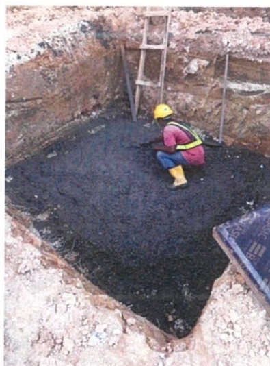
Figure 7: Pour crusher run and lean concrete
