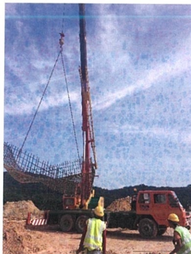
Figure 9: installing steel bar reinforced concrete pad footing
