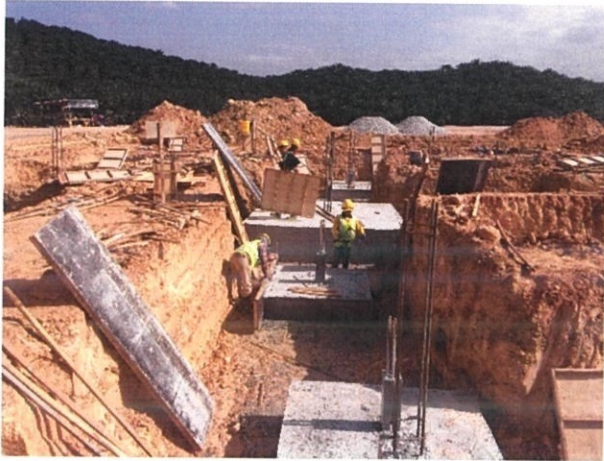
Figure 12: Dismantle formwork
