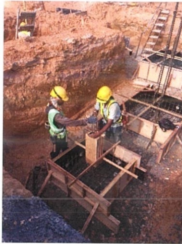
Figure 8: Installing formwork reinforced concrete pad footing
