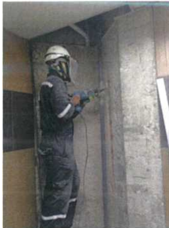
Figure 3.11 Worker wear face shield during hacking work
