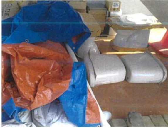
Figure 3.10 Material arrangement and cement stored
