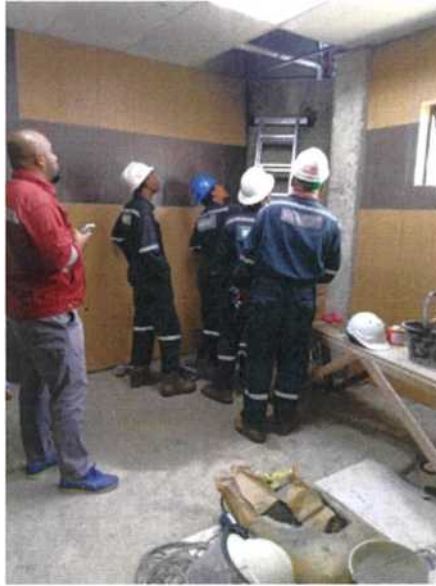
Figure 3.2 Inspection by Safety Officer during plumbing work
