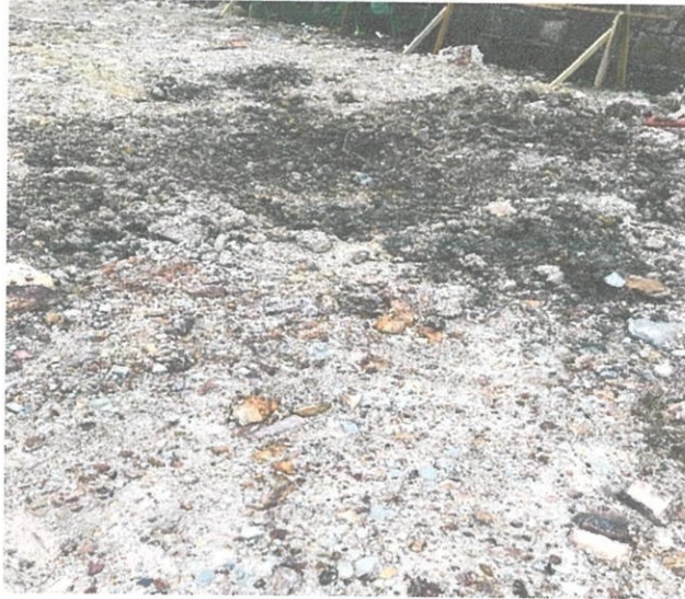
Figure 3.4: the hole was dig with area of 2ft x 2ft and depth is 6inch.
