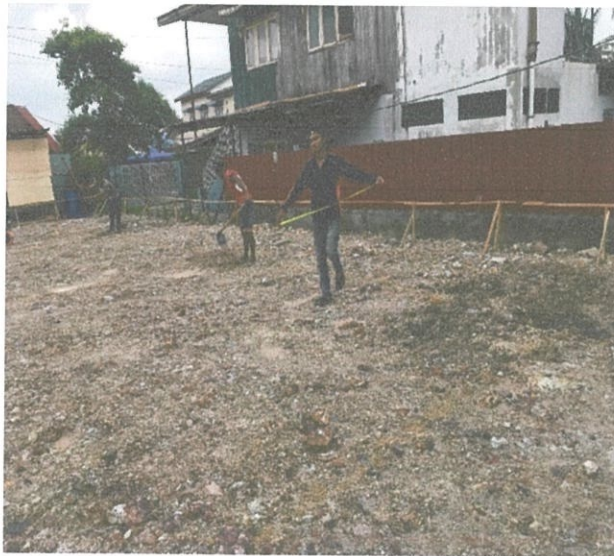
Figure 3.3: Marking the area of pad foundation and the area of house.
