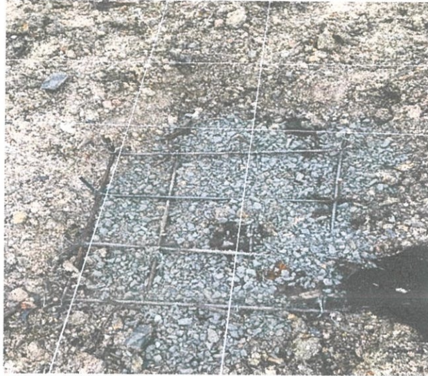
Figure 3.6: lay some coarse aggregate
