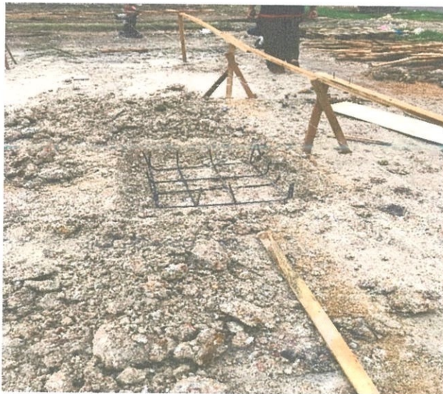
Figure 3.5: the reinforcement bars was place in the hole
