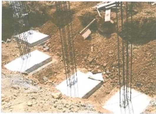
Figure 3.2 pad foundation
