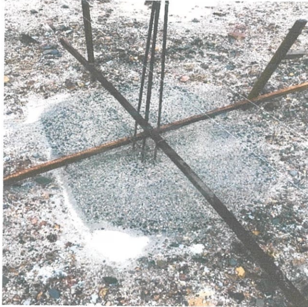
Figure 3.8: concrete the foundation.
