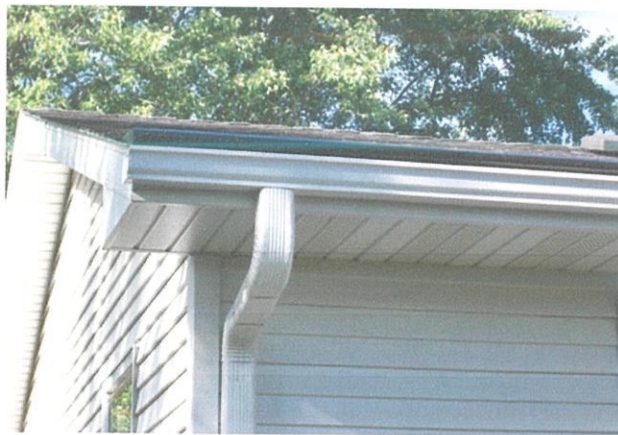
Figure 3.10: gutters at the roof
