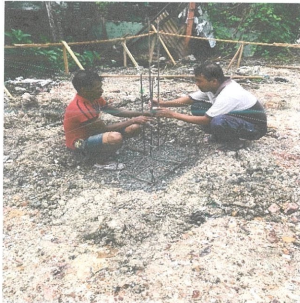
Figure 3.7: the reinforcement bars are tied to make a connection
